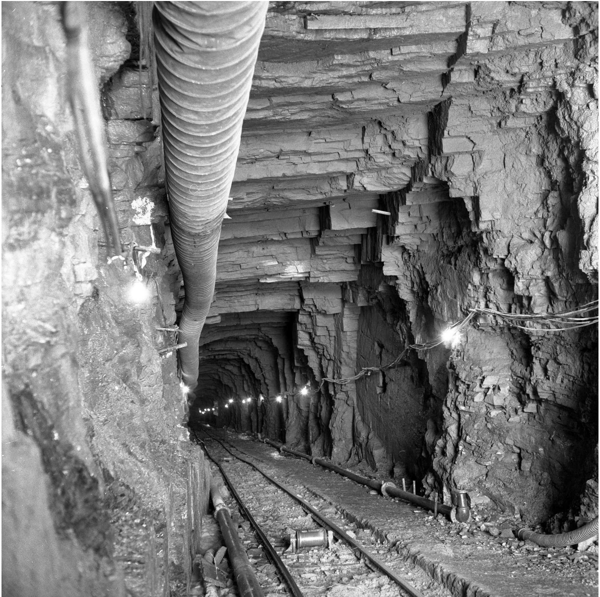
Fig. 2.9 Photograph at an unknown locality within the LEDT to demonstrate the relationship between the shallowly dipping (bedding) planes intersecting the steeply dipping (joint) planes that are related to faulting
