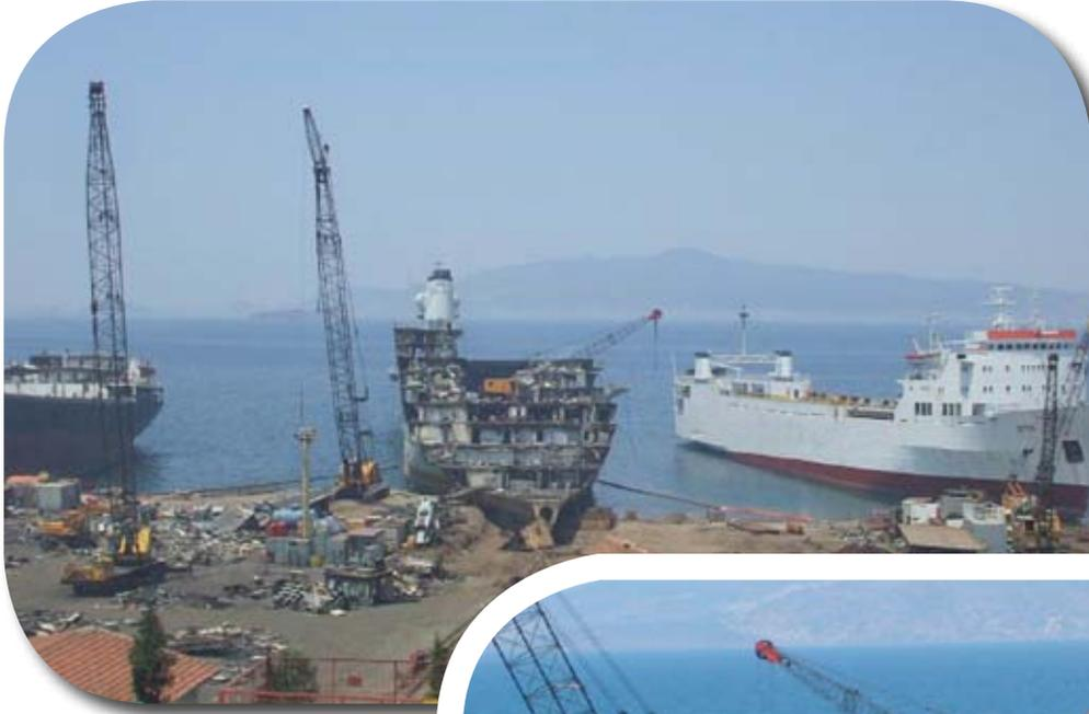
Progress of works showing dismantling of superstructure
