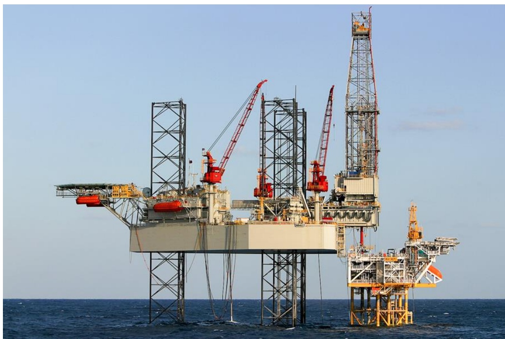
Figure 3.1 – Typical jack-up rig (e.g. shown is the Ensco 104) over a small platform
