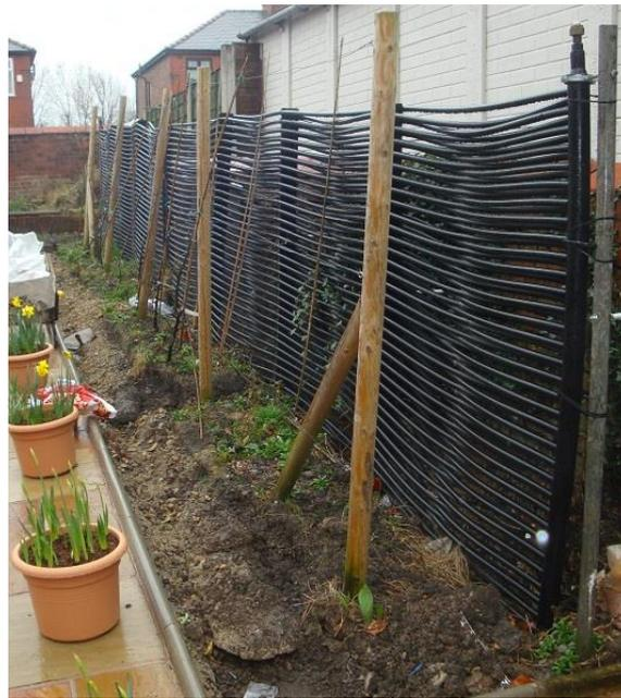
Figure T 21 – “Energy Fence” installed in garden of house
