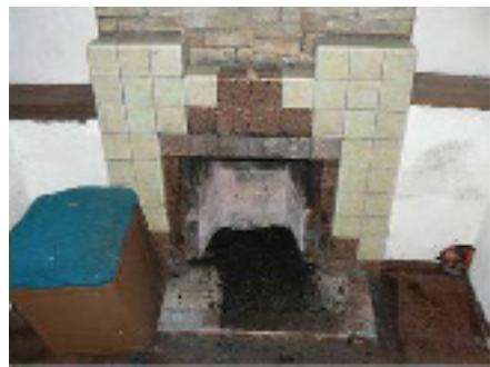
**Fire hazard – open fireplace:** with no barrier to prevent hot coal and ashes falling onto the carpet.
