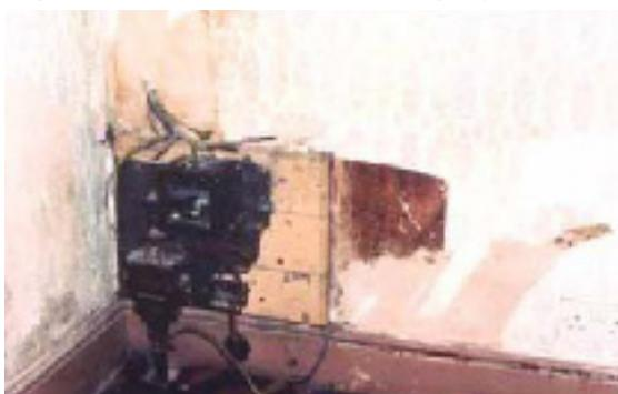
**Old wiring and sockets:** a number of which look damaged.
