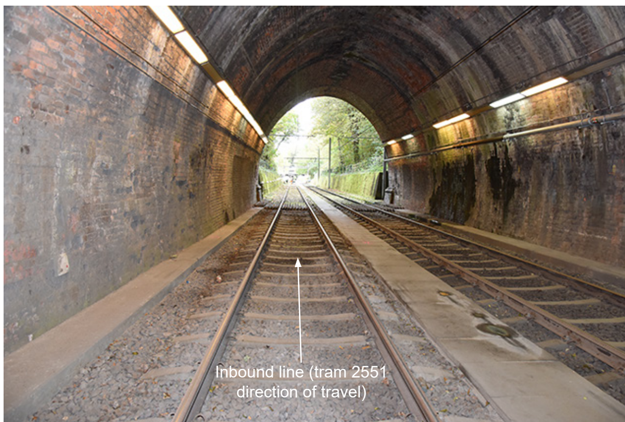
Figure 7: View towards Sandilands south curve from within the third tunnel
