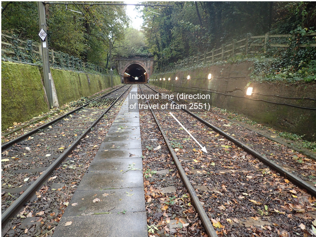
Figure 20: Inbound line between tunnels and speed sign six and a half hours after the accident. No evidence of significant leaf contamination on the rail head.
