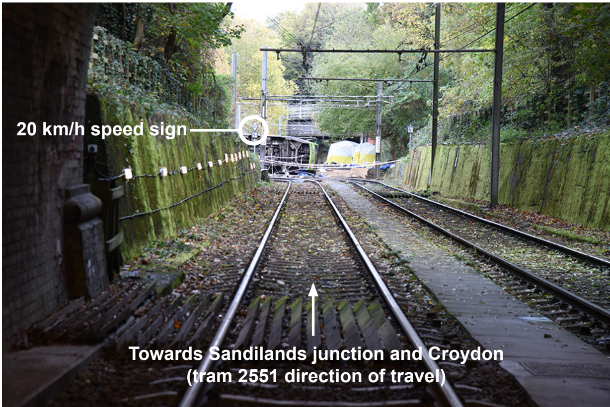
Figure S1: View emerging from the tunnels
