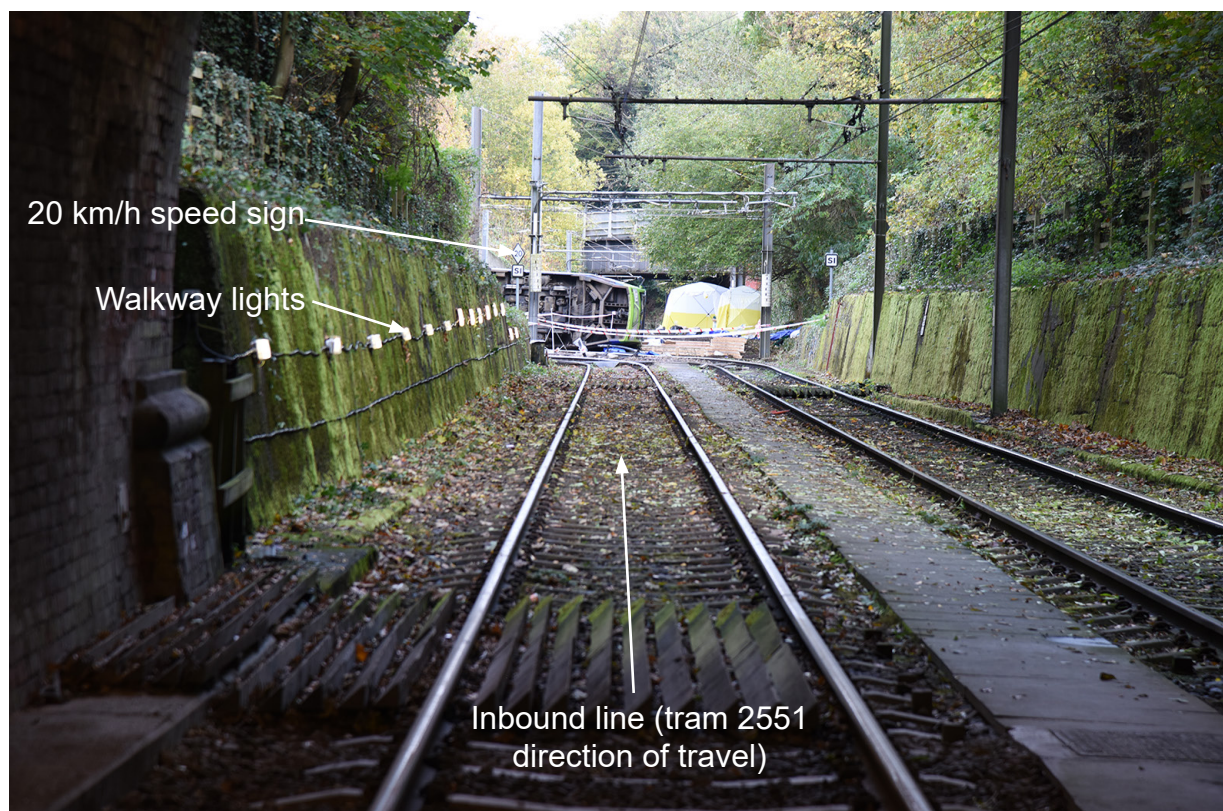
Figure 9: Approach to Sandilands south curve viewed from tunnel exit (overturned tram visible in distance)
