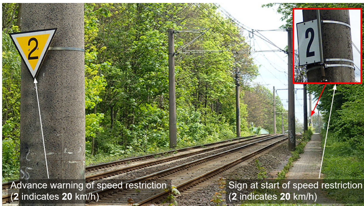
Figure 29: BOStrab advance warning of speed restriction on the Cologne tramway
