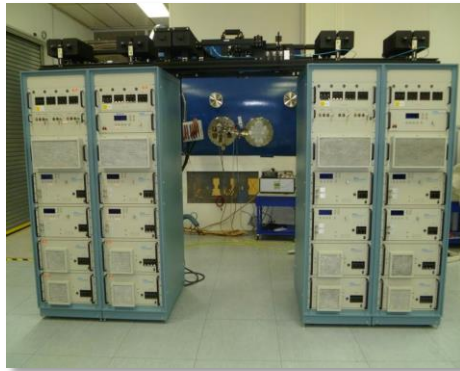
Figure 3.16 High power Ku-band amplifiers
