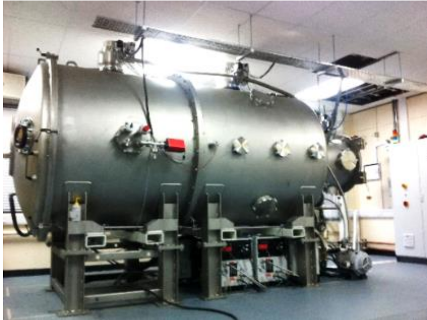
Figure 3.198 Thermal Vacuum Facility within the David Fearn EP Laboratory
