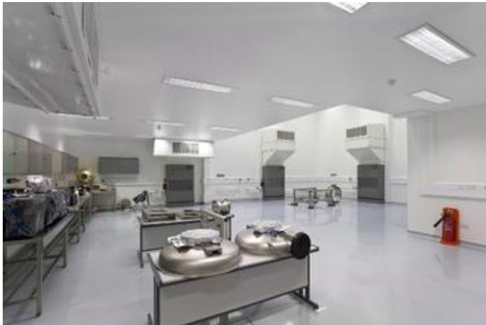
Figure 3.179 MSSL ISO-8 high-bay/low-bay clean room (left) and ISO-5 super-clean room (right)
