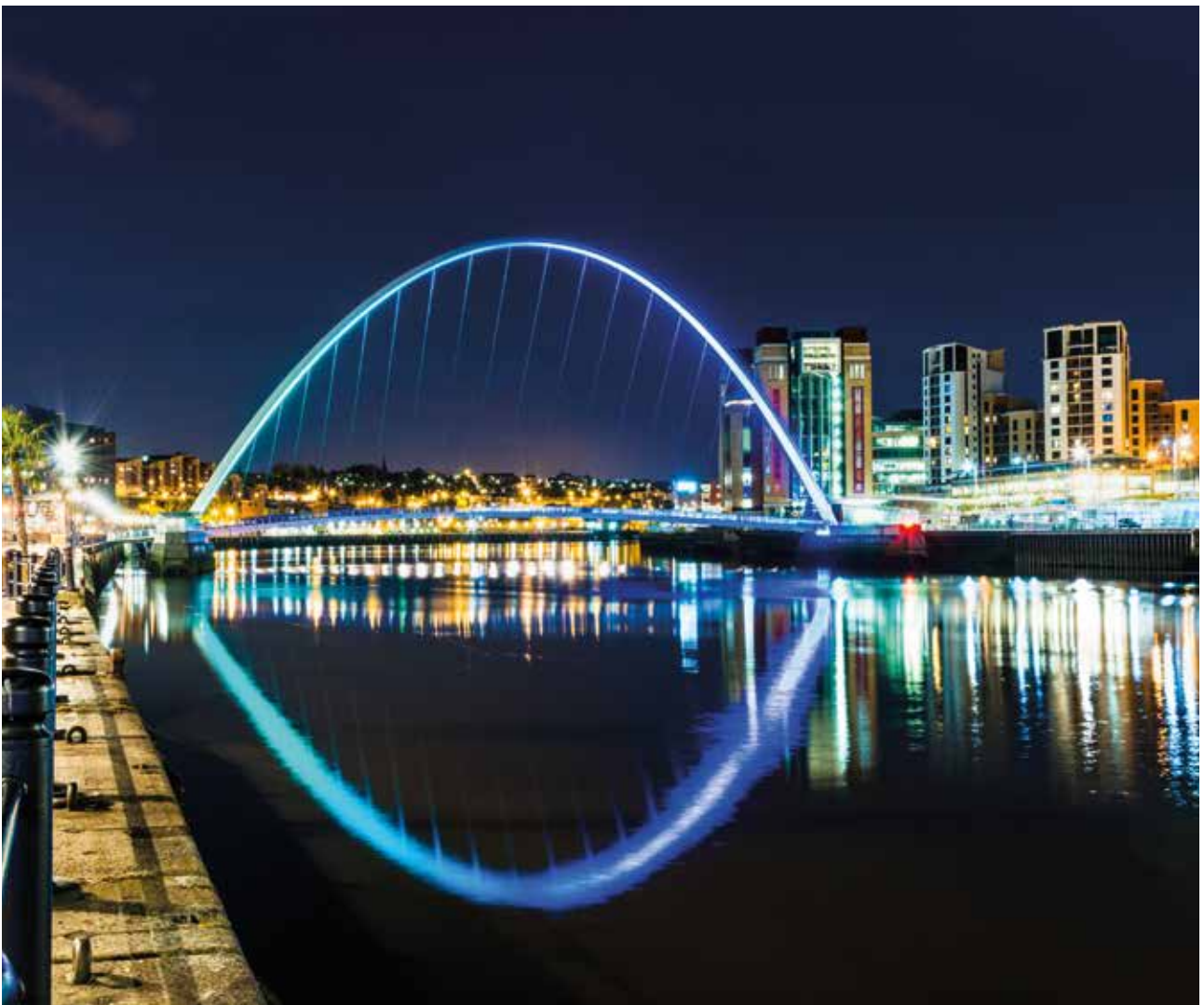
Gateshead Millennium Bridge, Newcastle
