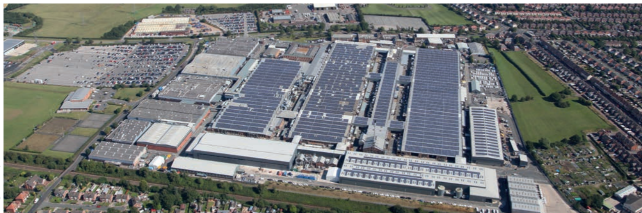
Bentley car production factory, Crewe
