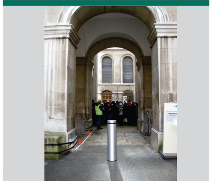
Figure 10: Bollard placed within exit opening (0m stand-off)
