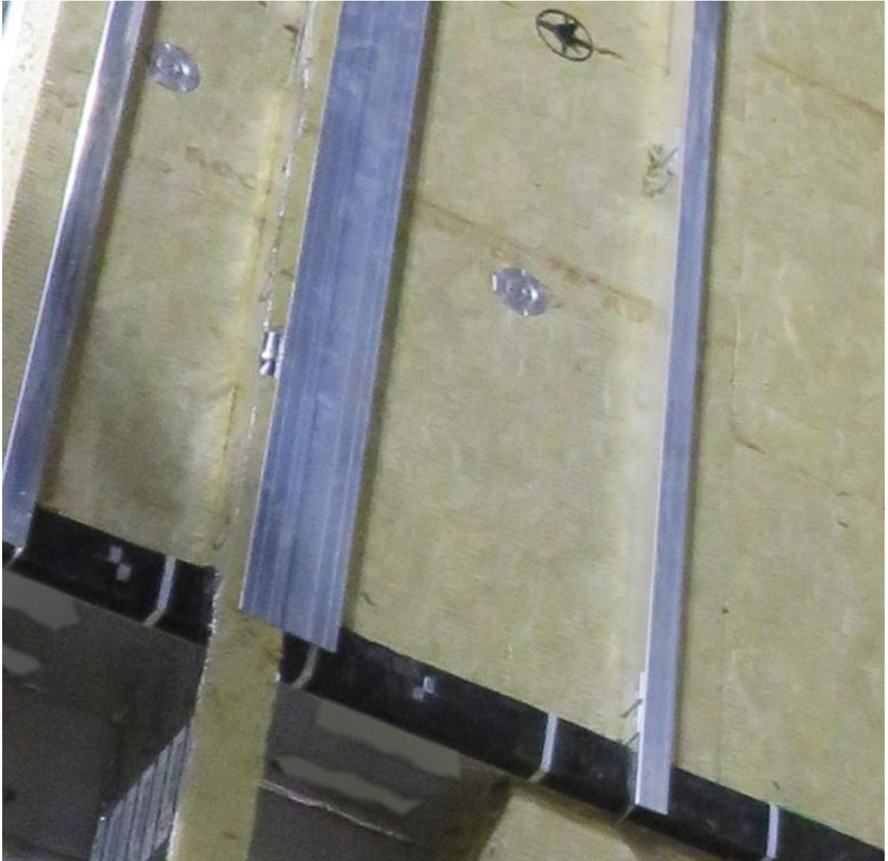
Figure 4. Horizontal intumescent cavity barrier fixed through the entire depth on face turned steel brackets, at the intersection with a vertical cavity barrier.
