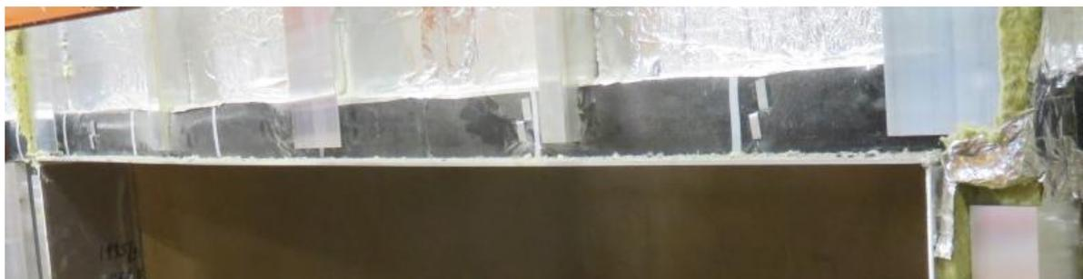
Figure 5. Horizontal intumescent cavity barriers fixed through the entire depth on face turned steel brackets, fitted above window pod.
