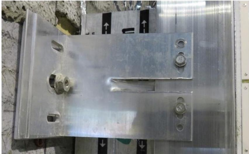
Figure 8. Example of aluminium rail fixed to 'L' bracket through movement holes.
