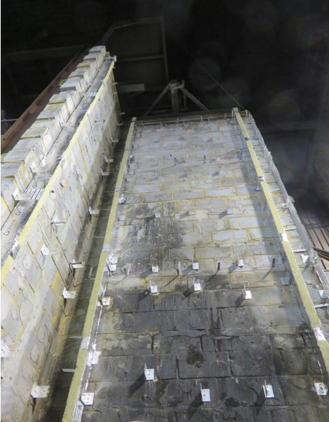
Figure 3. Location of 'L' brackets (partially visible) and vertical cavity barriers.
