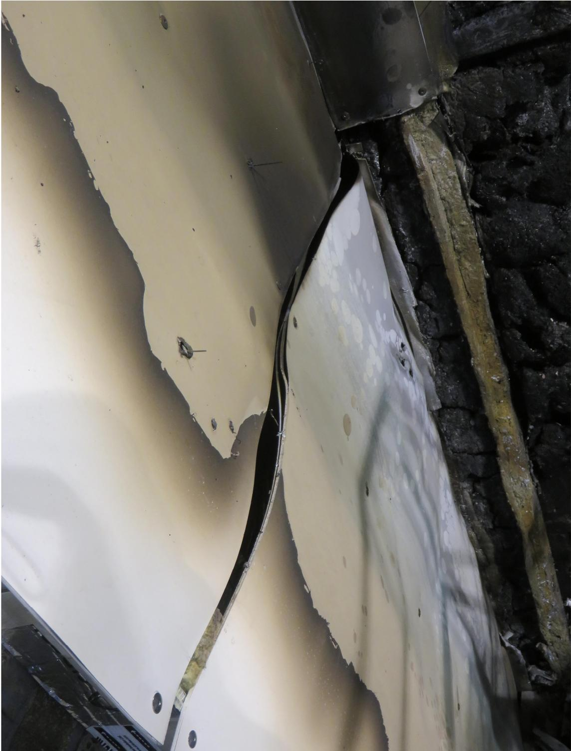
Figure 29. Distortion and delamination of ACM panel 1A – note some filler material remains intact.
