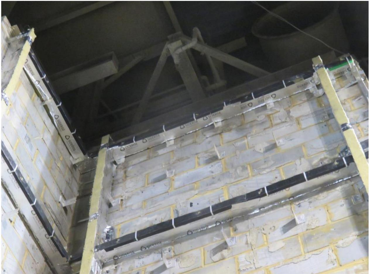
Figure 4. Horizontal intumescent cavity barriers fitted between vertical cavity barriers.
