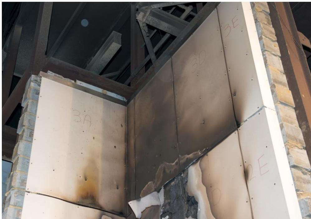
Figure 28. Third row ACM panels (approximately 4600mm-6500mm above combustion chamber).
