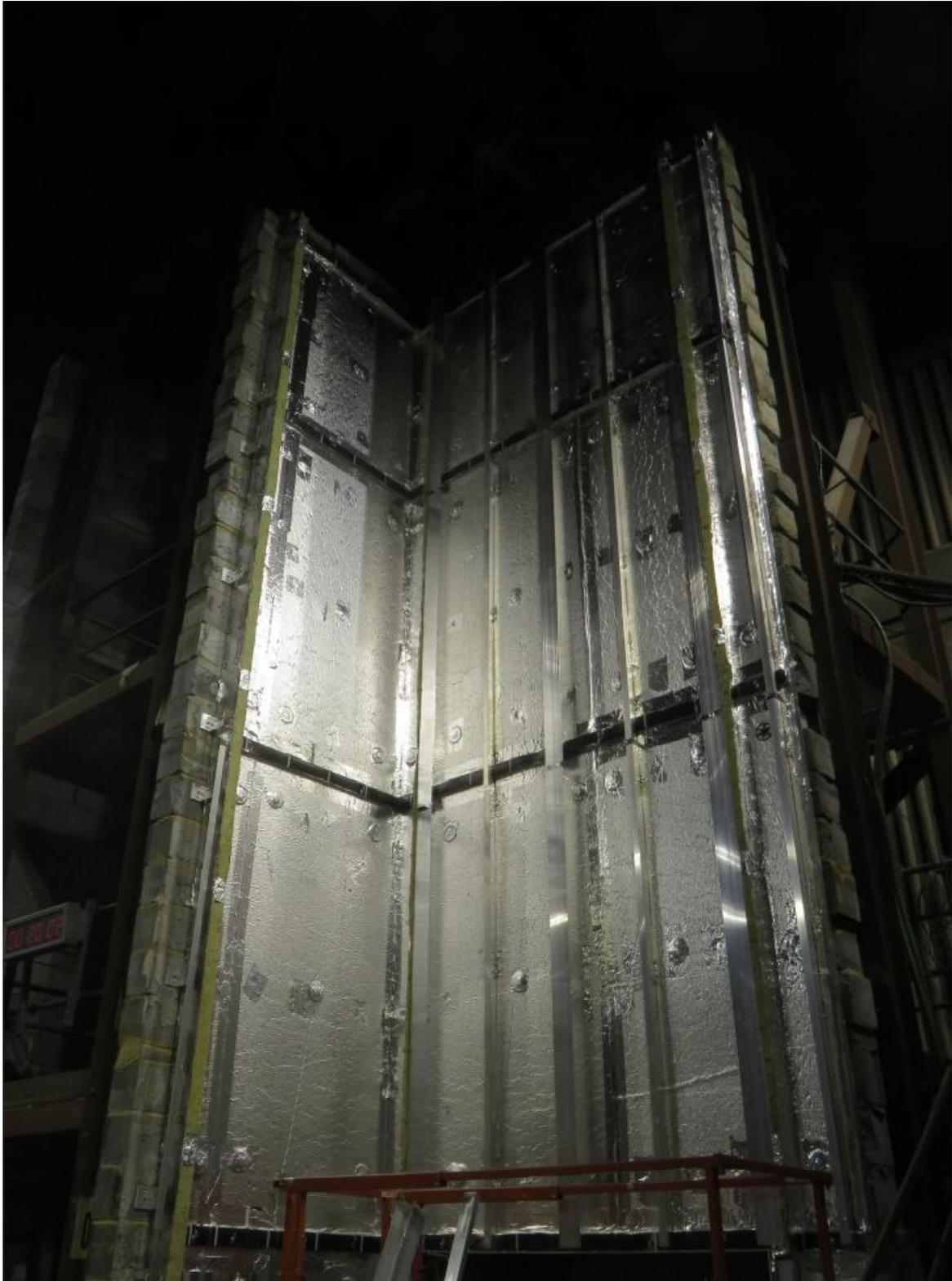
Figure 10. Completed installation of railing substructure visible on main wall.
