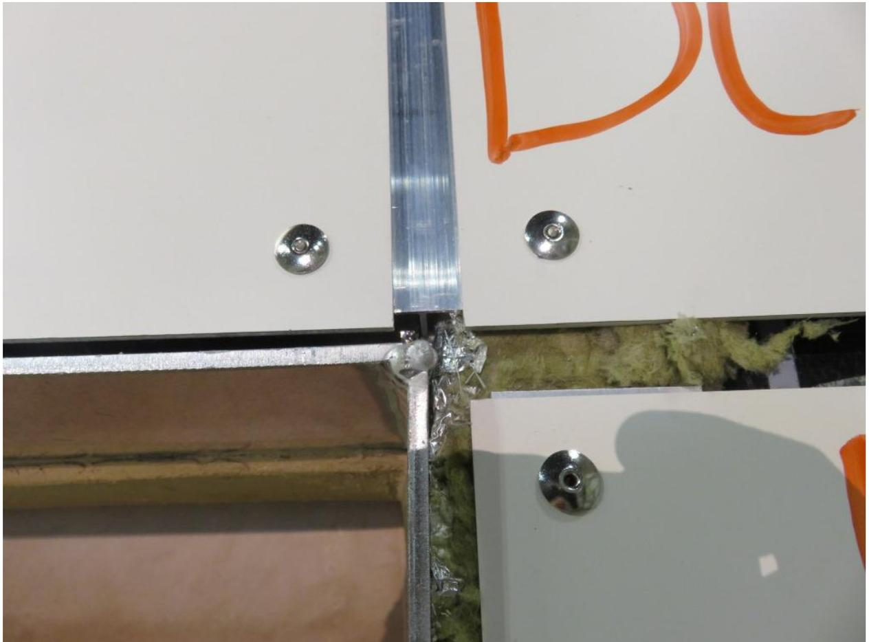
Figure 11. Detail at corner of combustion chamber opening. Panels riveted in place with nominal 20mm vertical gap for ventilation purposes.
