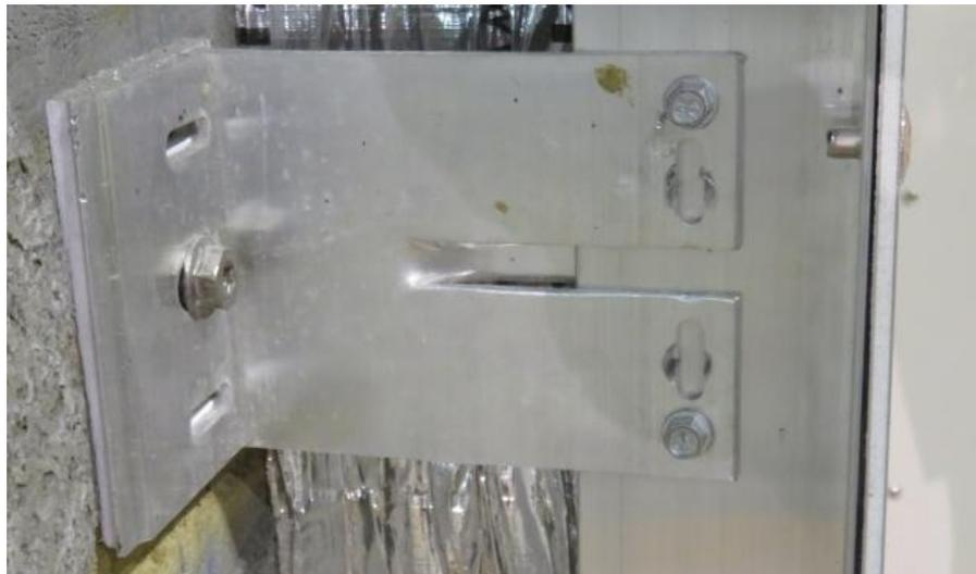
Figure 9. Example of aluminium rail fixed to 'L' bracket through fixed holes.
