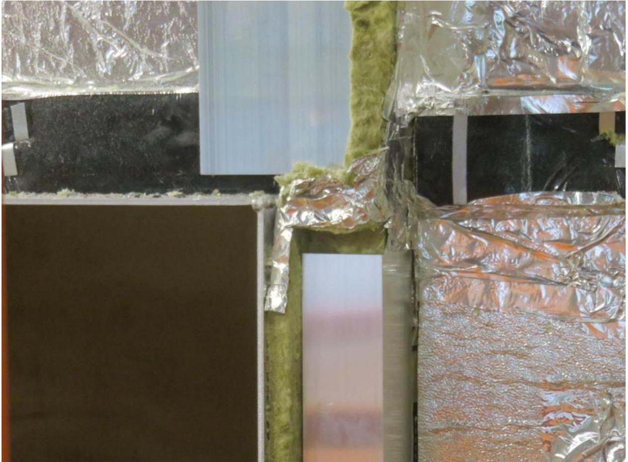
Figure 6. Vertical cavity barrier cut to fit under 'T'-rail.
