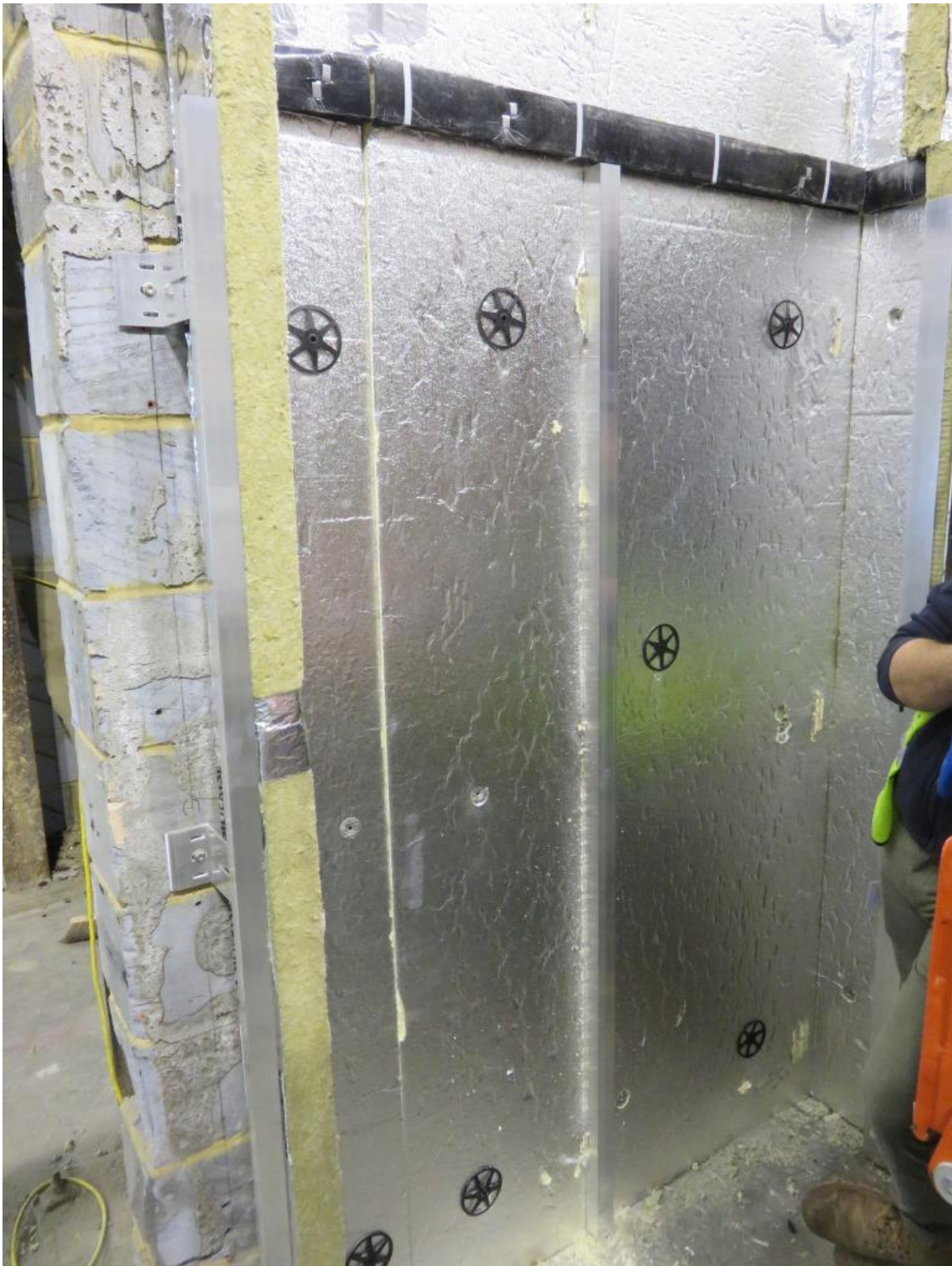
Figure 8. Insulation fixings applied and 'L'-rail embedded into panel.
