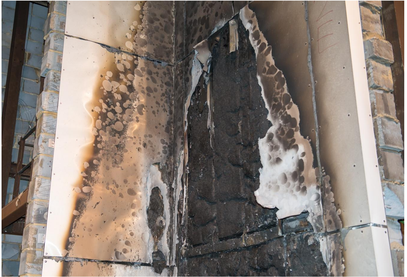
Figure 27. Second row ACM panels (approximately 2300mm-4600mm above combustion chamber).
