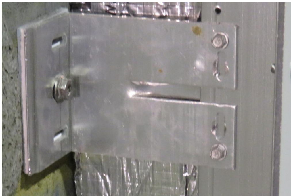
Figure 11. Example of aluminium rail fixed to 'L' bracket through fixed holes.
