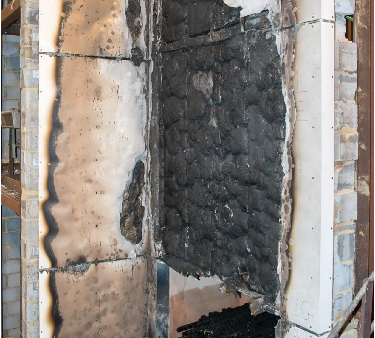
Figure 26. First row ACM panels (directly above combustion chamber).
