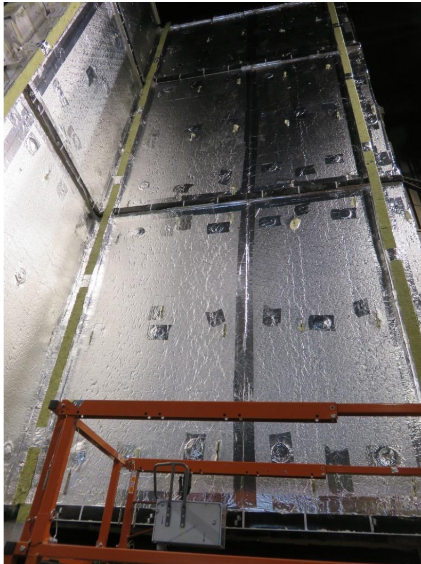
Figure 9. Joints and fixings covered with aluminium tape.
