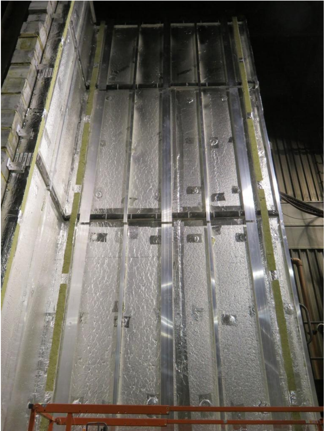
Figure 12. Completed installation of railing substructure visible on main wall.
