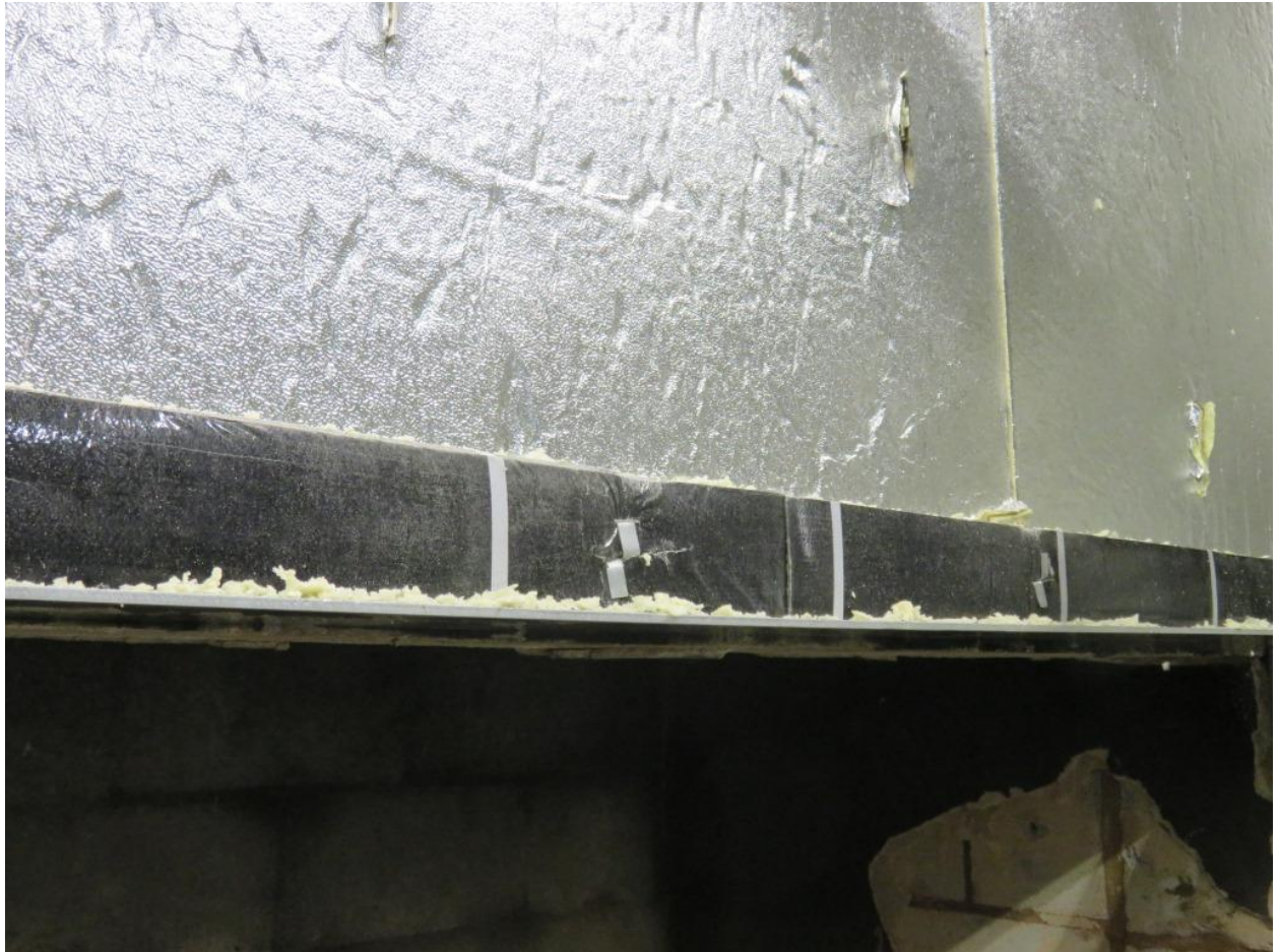
Figure 6. Installed window pod lining combustion chamber.
