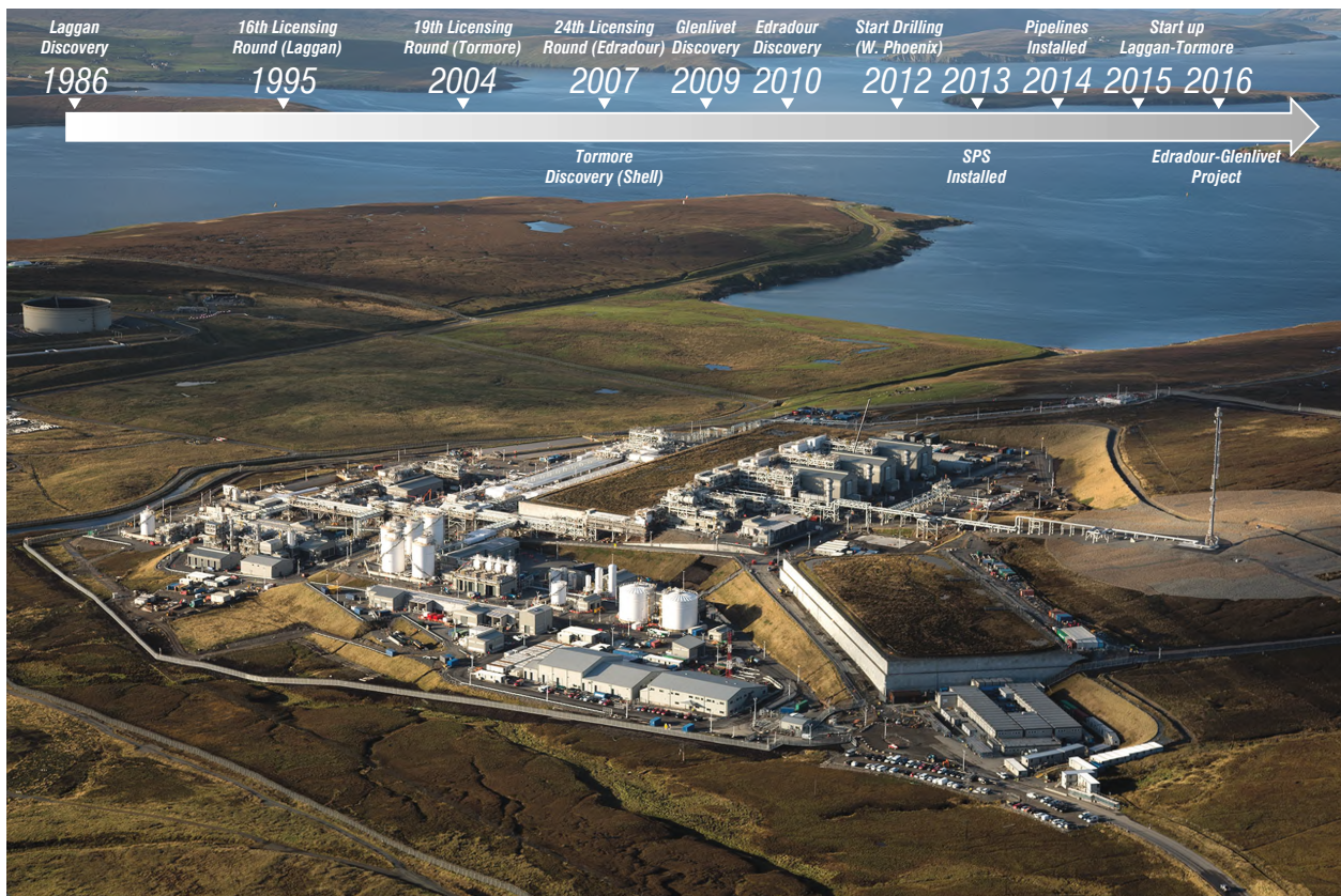
Figure 7 : The Shetland Gas Plant
