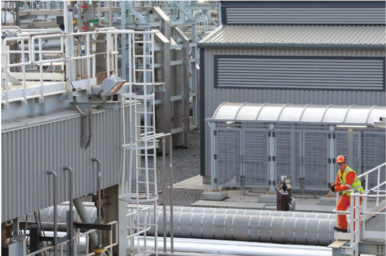
Figure 2 : Operations at the Shetland Gas Plant
