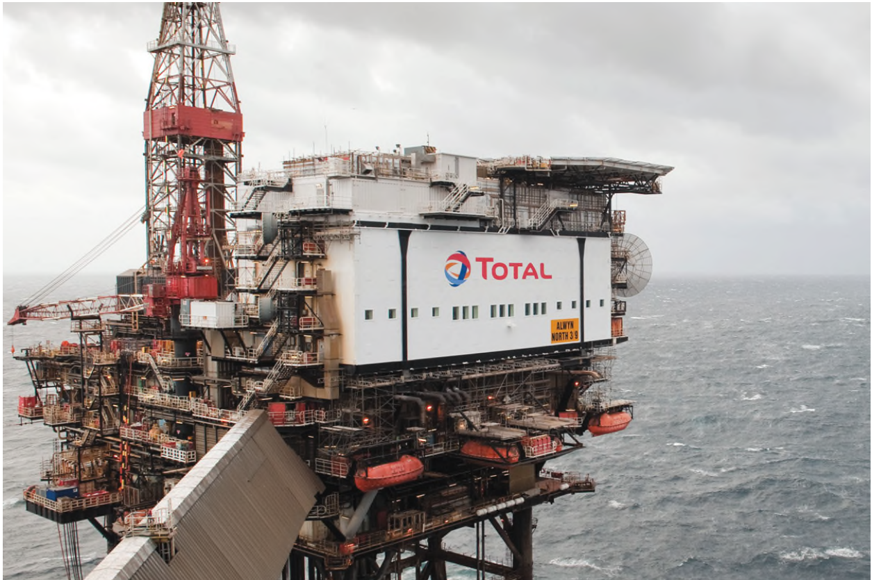
Figure 4 : Alwyn North Platform
