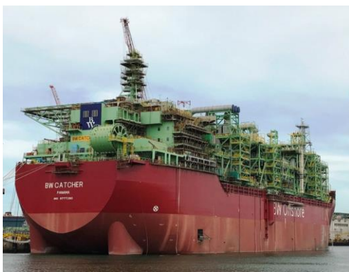
Figure 2.11 – Catcher FPSO in construction
