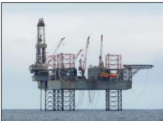
Figure 2.15 – Ensco 100 Drilling Rig
