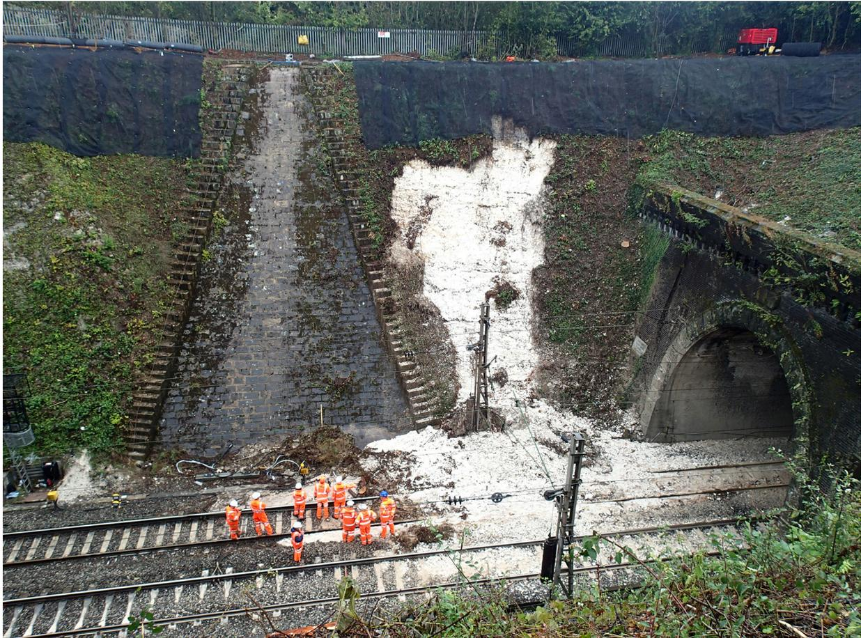
Figure 5: View of landslide and debris on track. The adjacent masonry structure is a face wall (refer to paragraph 90).
