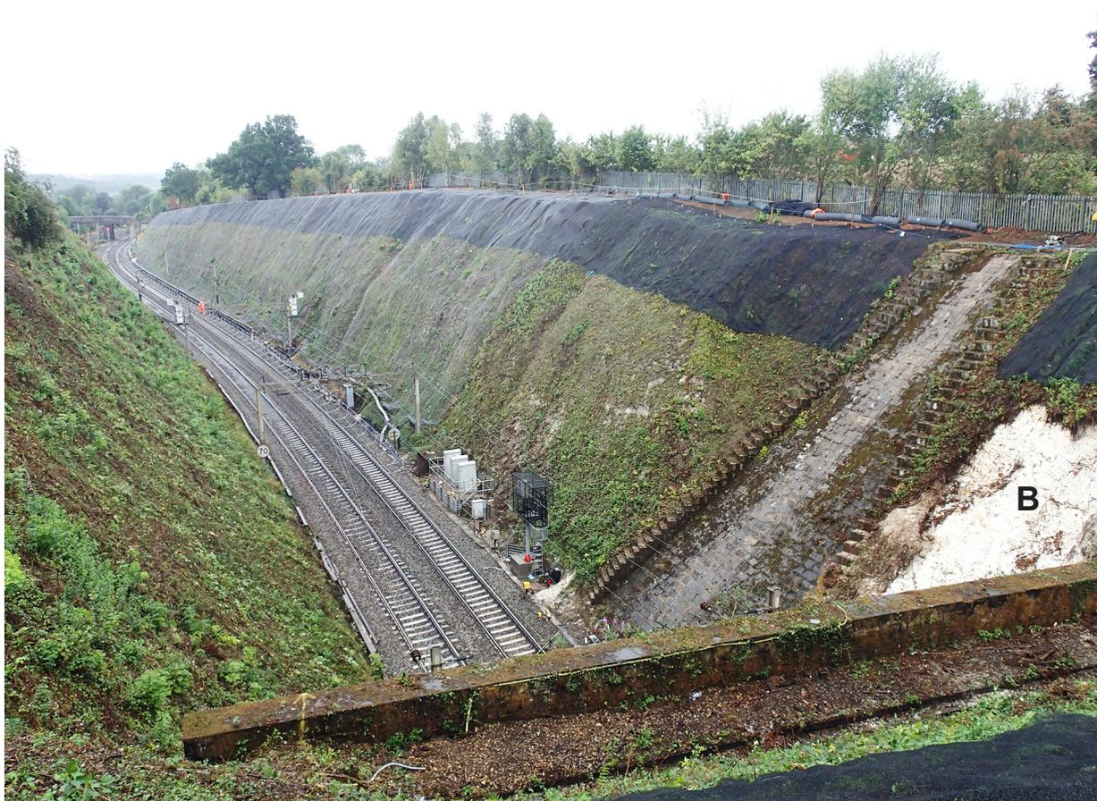
Figure 7: View of slow lines cutting from above tunnel portal, looking north-west towards Gypsy Lane bridge on 16 September 2016. The partly completed slope protection works are visible. The landslide is marked 'B'.
