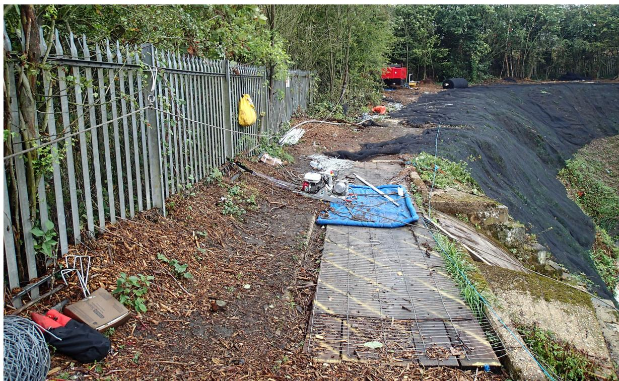
Figure 13: Concrete raft above face wall. Scaffolding boards had been placed inside the raft to remove a tripping hazard during the slope protection works.
