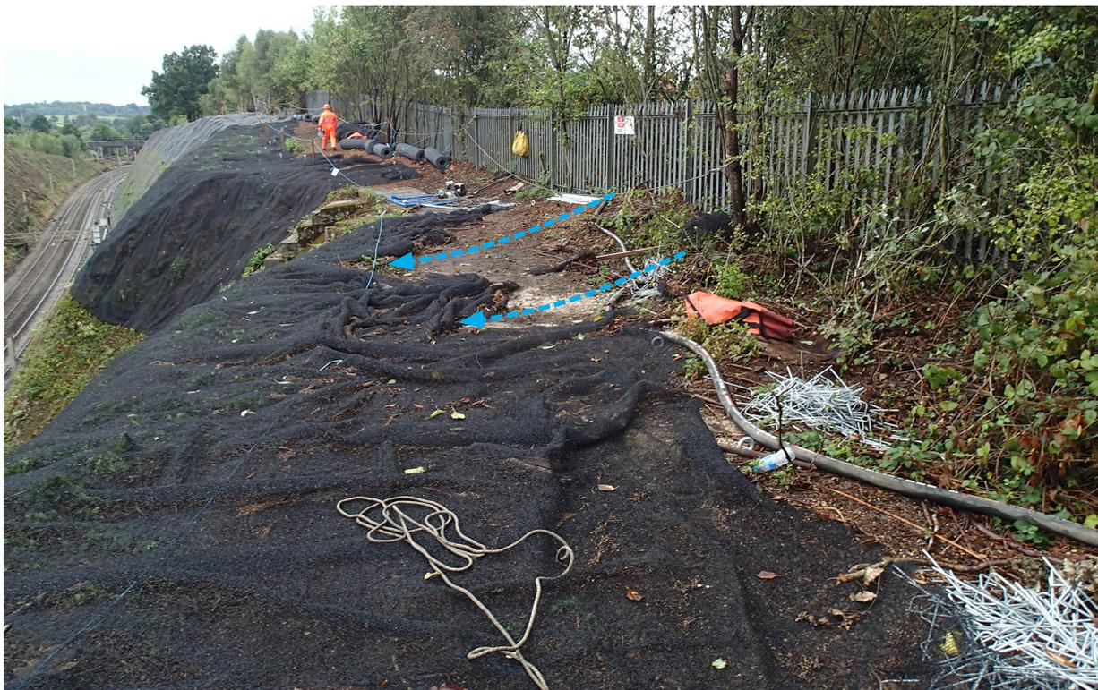
Figure 9: Crest of cutting above landslide showing erosion matting displaced by surface water flow
