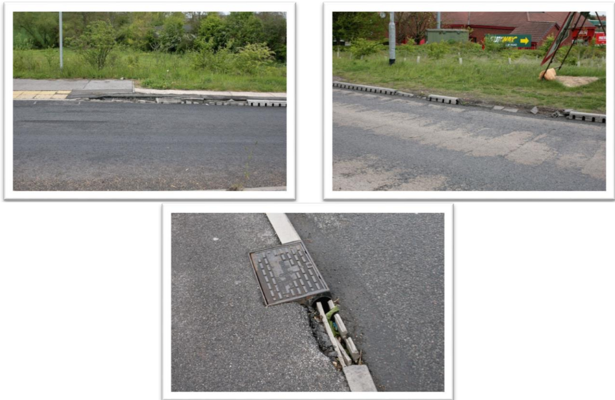
Figure 5.27 – Damage to the kerb drainage system at the two locations on the northbound entry-slip road/ roundabout (top left and top right), and at the entrance to the southbound service area (lower centre) at Markham Moor.
