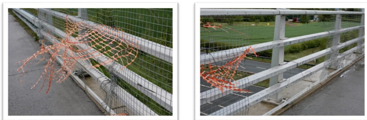
Figure 5.39 – Damage to the pedestrian parapet above the northbound carriageway on the overbridge at Carpenters Lodge.
