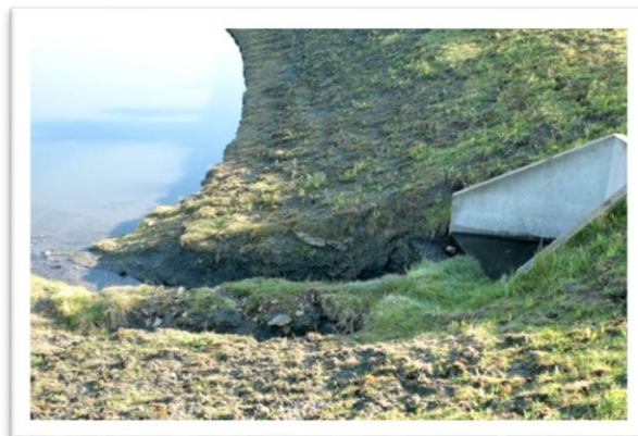
Figure 5.32 – Erosion at the inlet/ outlet of the balancing pond to the southwest of the junction at Gonerby Moor.
