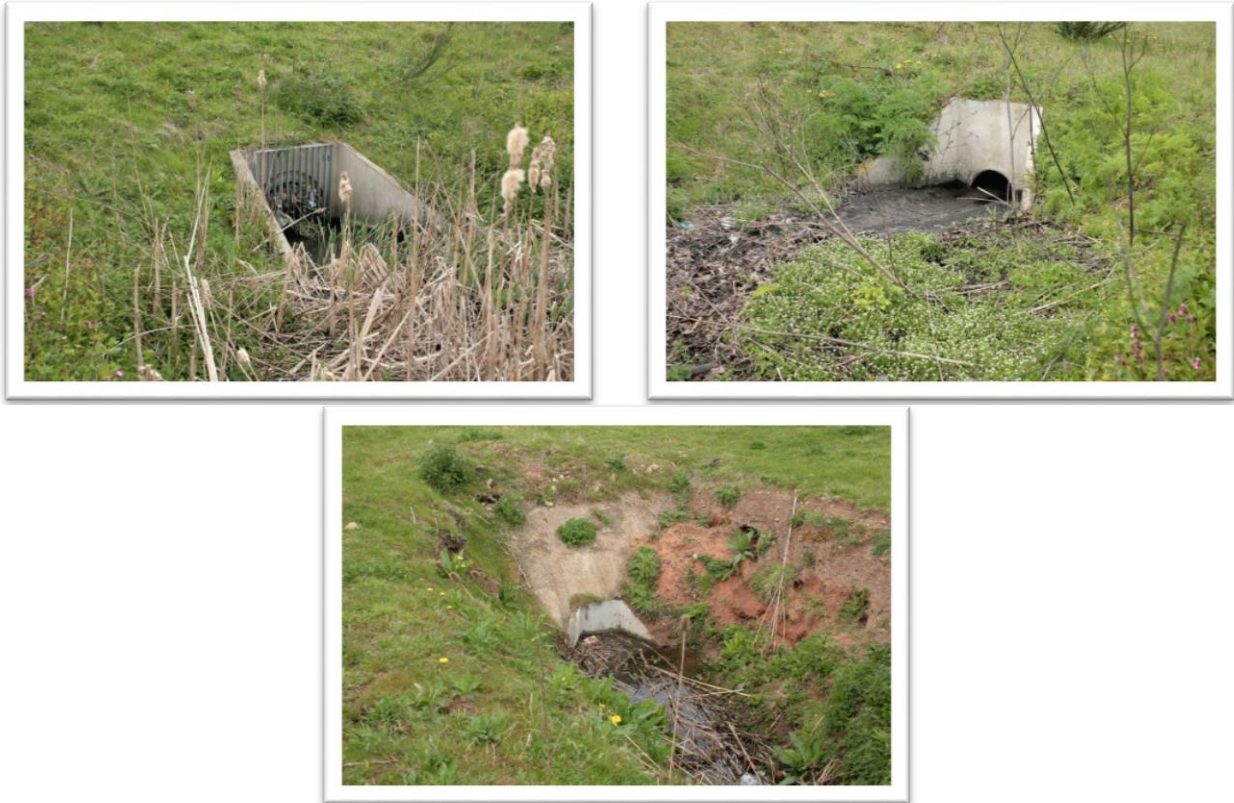
Figure 5.24 – Ponding evidence in the form of silt build-up at the entrance to Whitewater Lane from the southern roundabout at Blyth. Partially blocked inlets/ outlets at the southern balancing pond at Apleyhead (top left) and adjacent swale (top right), and standing water at the swale adjacent to the northbound carriageway, just south of the overbridge (lower centre).
