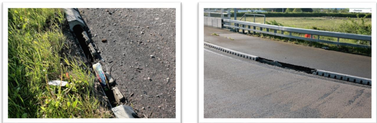
Figure 5.31 – Damage to the kerb drainage system at the western roundabout at Gonerby Moor.
