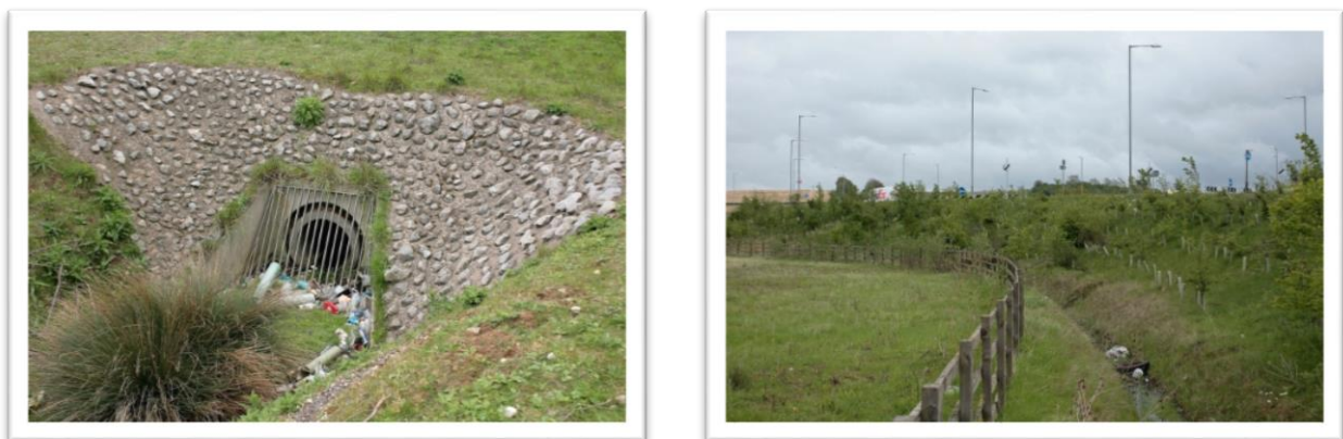
Figure 5.28 – Litter build-up within the drainage system at Markham Moor, adjacent to the southbound entry-slip road (left), and at the A57 junction with the northern roundabout (right).
