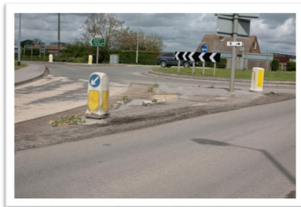
Figure 5.38 – Silt and debris partially obscuring the tactile paving on the NMU route at the roundabout to the northeast of the overbridge at Colsterworth south.
