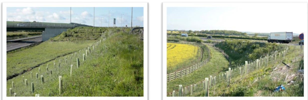
Figure 5.2 – Large areas of new planting flanking the northbound entry-slip road at Gonerby Moor.
