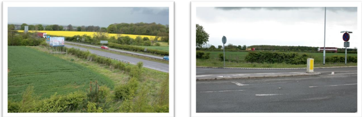
Figure 5.15 – Although the newly planted hedgerows are generally developing as expected (either side of the carriageways north of the Carpenters Lodge overbridge (left), a significant section of the translocated hedgerow appears to have failed (right).
