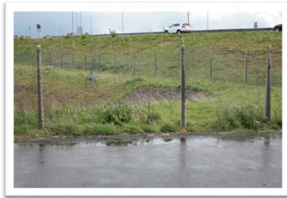
Figure 5.30 – The breached fence enclosing the balancing pond adjacent to the access road/ car park of the Chinese restaurant at Markham Moor.
