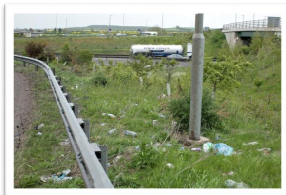
Figure 5.9 – A significant quantity of litter was observed between the northbound entry-slip road and the northbound carriageway at Markham Moor.
