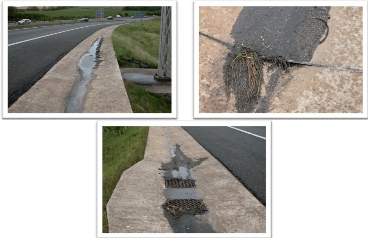
Figure 5.29 – Ponding within the drainage system at Markham Moor, adjacent to the northbound exit-slip road (top left) caused by detached drainage unit joints (top right), and silt/ vegetation building up at the protective grilles on the drains at the same location (lower centre).
