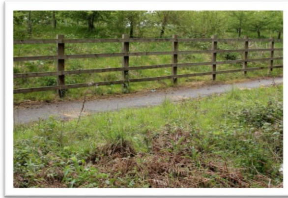
Figure 5.34 – A tarmac, rather than gravel, surface has been provided along the bridleway adjacent to the northbound exit-slip road at Apleyhead.
