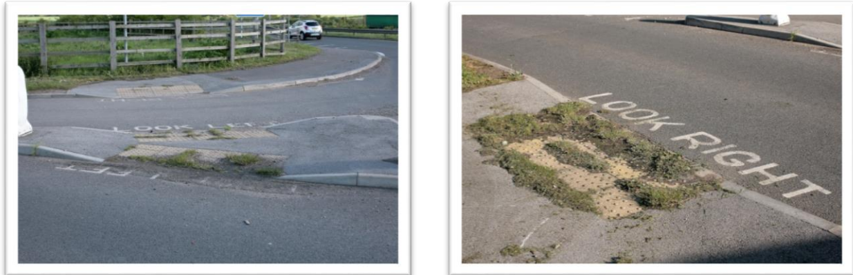
Figure 5.23 – Ponding evidence in the form of silt build-up at the entrance to Whitewater Lane from the southern roundabout at Blyth.
