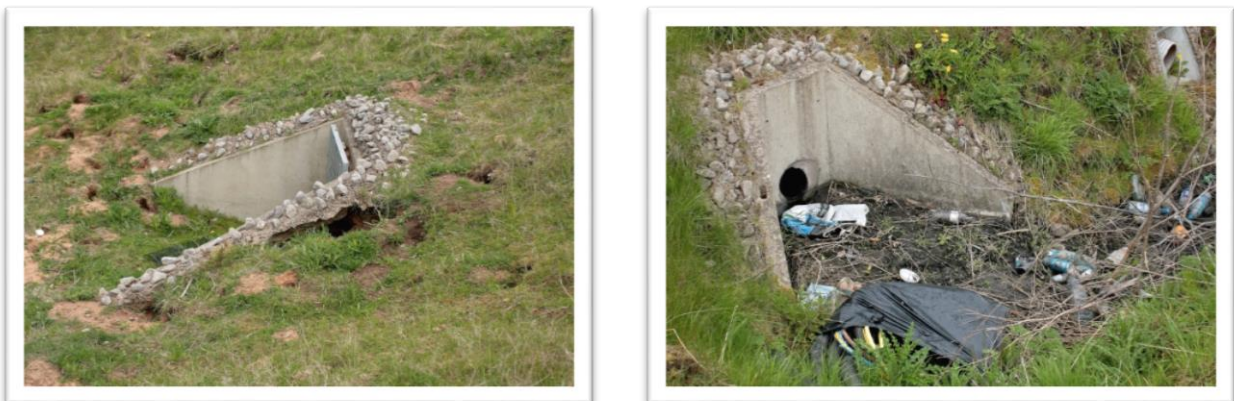
Figure 5.25 – Damage to the inlet/ outlet at the northern balancing pond (left), and litter/ silt building up near the roundabout to the east (right) at Apleyhead.
