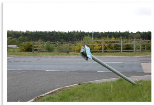
Figure 5.36 – Damaged NMU signage opposite the western corral at Apleyhead.
