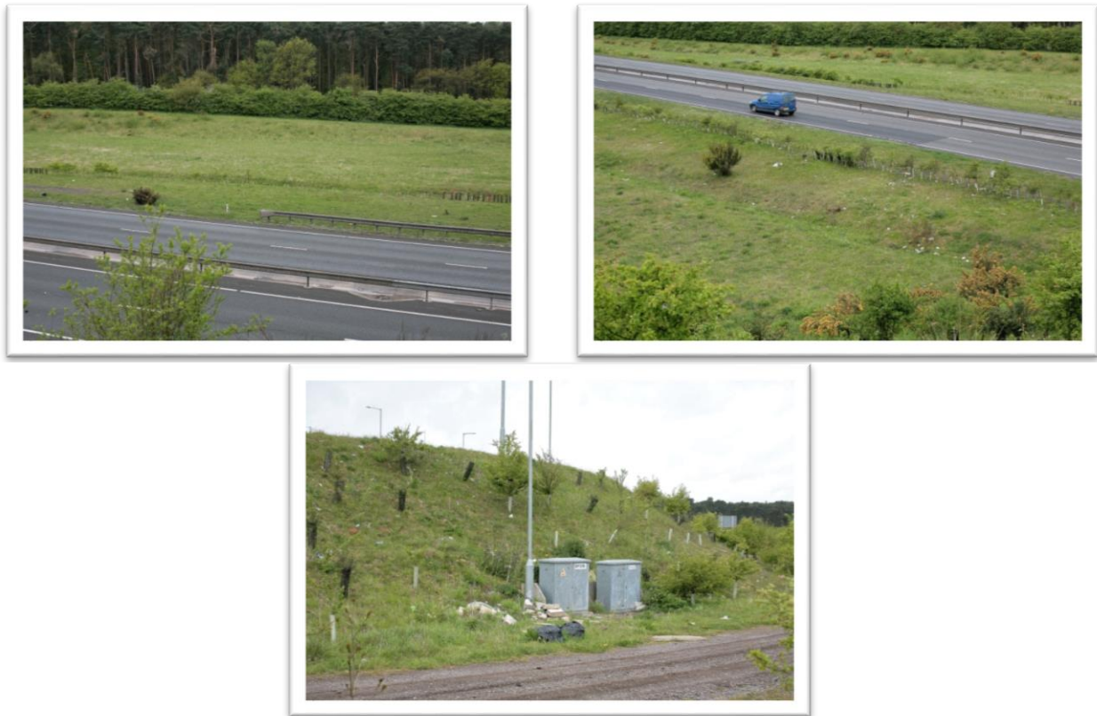
Figure 5.7 – The hedgerows south of the Apleyhead overbridge adjacent to the northbound (top left) and southbound (top right) carriageways are performing significantly worse than expected, as is the planting plot adjacent to the bridleway at the eastern roundabout (lower centre).
