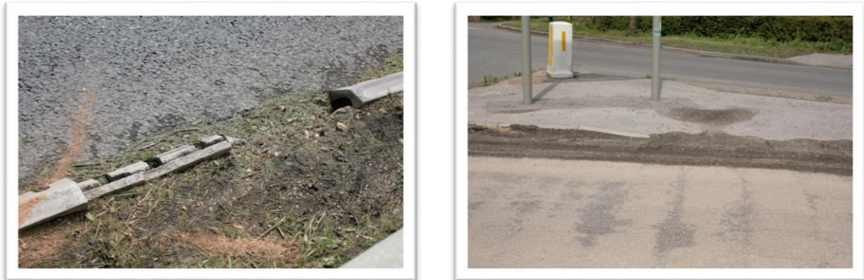
Figure 5.33 – Damage to the kerb drainage system at the roundabout to the northeast of the overbridge at Colsterworth south.
