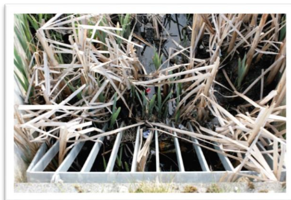
Figure 5.22 – Vegetation encroaching on the balancing pond inlet/ outlet grille at Blyth.
