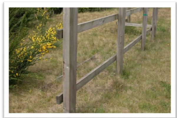
Figure 5.35 – The western corral at Apleyhead, showing the vegetation within (left) and the dislodged rail (right).
