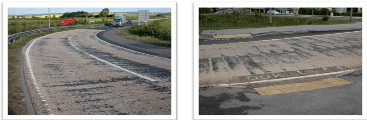
Figure 5.40 – Worn High Friction Surfacing on the southbound exit-slip road at Blyth (left), and on the approach to the A638/ A57 roundabout at Markham Moor (right).
