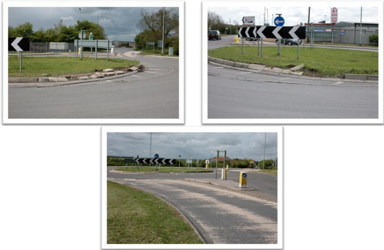
Figure 5.41 – Damage to the roundabouts at Colsterworth south: at two locations on the roundabout to the east of the A1 (top left and top right), and at the roundabout to the west of the A1 (lower centre), where it can also be seen that HFS on the approach to the roundabout is significantly worn.
