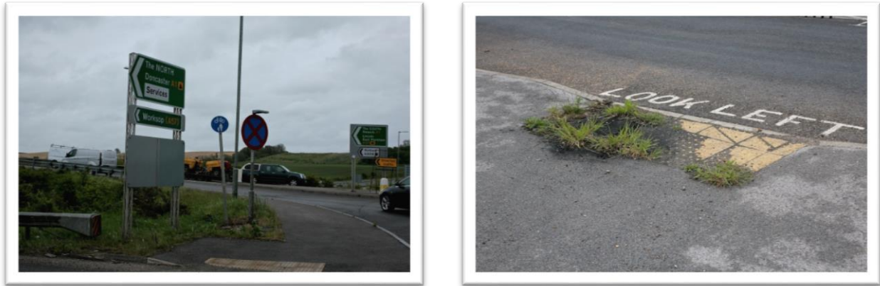
Figure 5.37 – The NMU directional sign at the eastern roundabout adjacent to the northbound entry-slip road at Markham Moor (left), and silt build-up partially obscuring the tactile paving at the same location (right).
