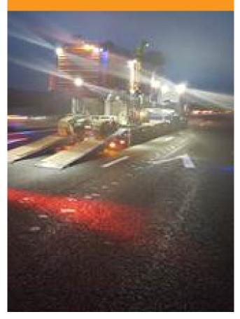
On the Manchester Smart Motorways Project, Aggregate Industries have developed a novel way of highlighting the restricted zones around their plant. As much of their work is undertaken at night, to ensure the limits of the zone is easily identifiable, coloured lighting is used to create the zone limits. So far this has proven to be a great success and Al's are looking at introducing this on all their pavers and other large plant items.
