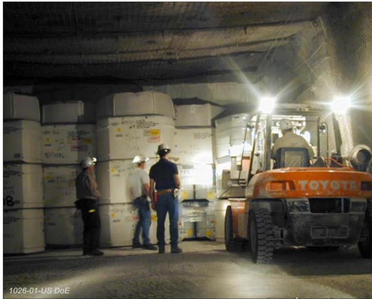
Figure 33 Contact-handled TRU waste packages being stacked in a disposal room in the WIPP with sacks of magnesium oxide backfill placed on top of the waste packages.
