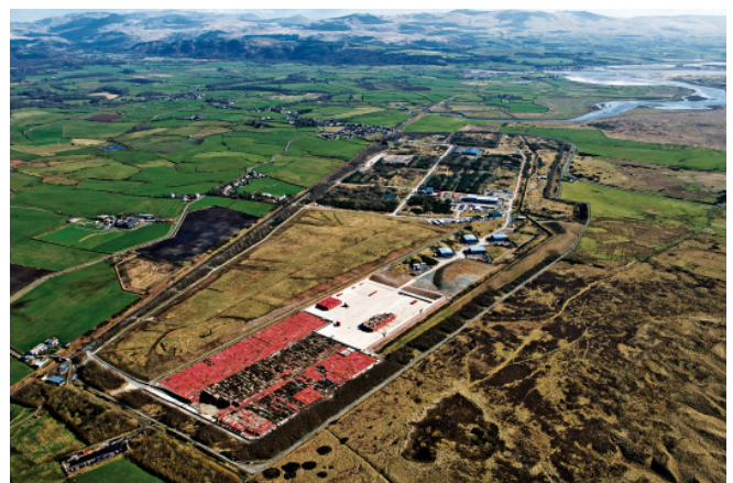
An aerial view of the LLW Repository near Drigg, Cumbria
