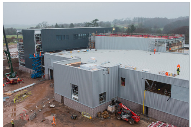
The CNC training facility underconstruction
