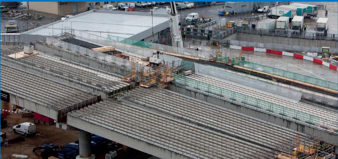
Picture: Precast concrete beams for multi-storey car park ramp.
