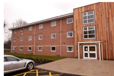
New Single Living Accommodation such as this SLAM development at Pirbright is improving the quality of life for military personnel
