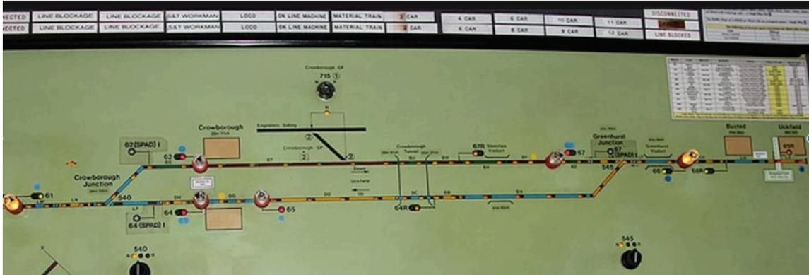
Oxtd Signalbox – Crowborough station layout, showing existing rarely used engineers siding in black controlled currently by a ground frame. Changes to the signalling would be desirable to enable the sidings to be used for regular empty train shunts and stabling, but not essential: a well maintained ground frame could enable access to the sidings until such time as the route signalling is renewed. A night-shift shunter would be required to operate the ground frame if it remained.
