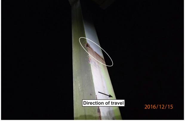
Figure 9: Witness marks (highlighted) on the gantry indicative of an earlier vehicle impact
