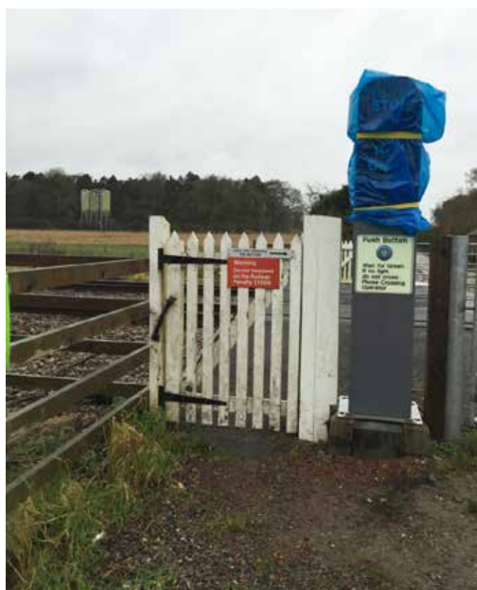
Figure 19: Decommissioned EBI Gate system – image taken on 08/12/2015 (Courtesy of Network Rail)
