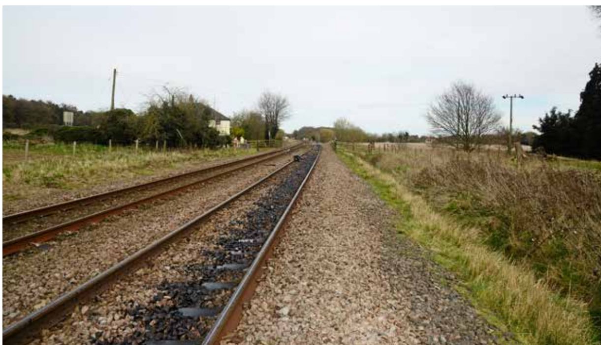
Figure 15: View from the rear of train 1K77 looking towards Hockham Road UWC
