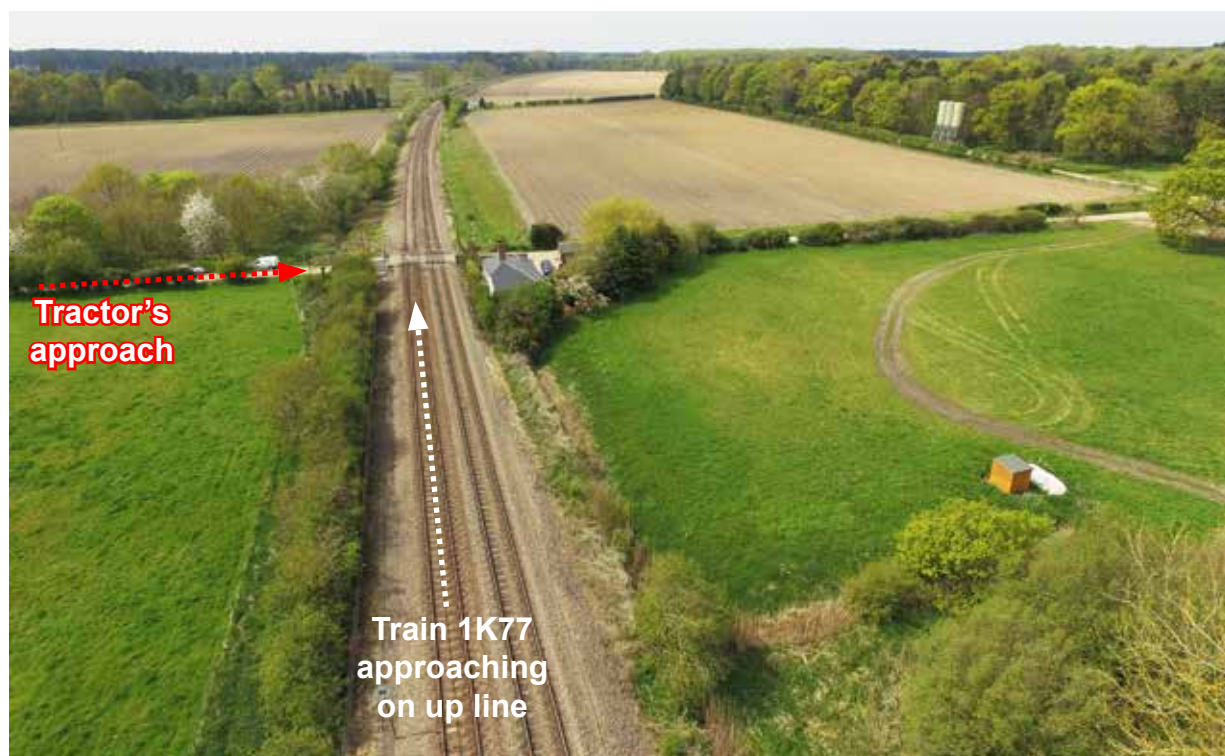
Figure 9: View looking towards Hockham Road UWC for trains approaching in the up direction
