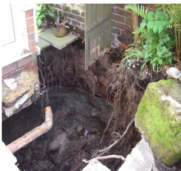
The collapse of shallow coal mining workings
