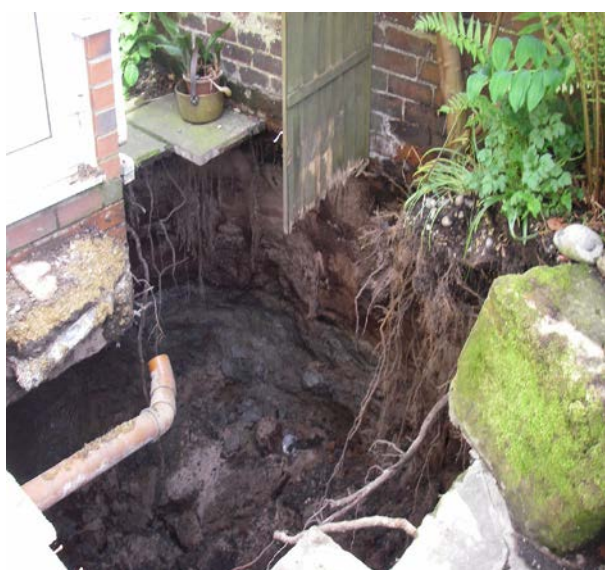
The collapse of shallow coal mining workings
