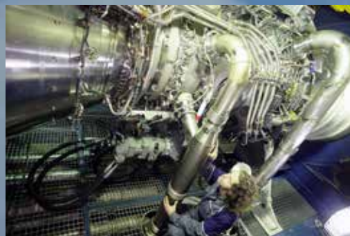
Above: Rolls-Royce oversee tests on the Type 26 MT300 gas turbine engine last February
