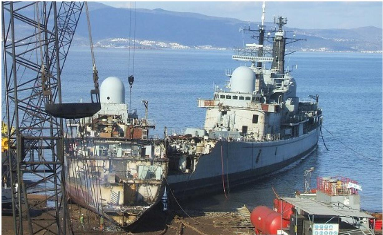
7 Jan 2016 – Ex-HMS Edinburgh in the foreground & Ex-HMS York in the background. Showing stages of pre-cutting ready for the hull to be winched up the dry slipway. Heavy Machinery is used to remove large pieces of the vessel for processing.
