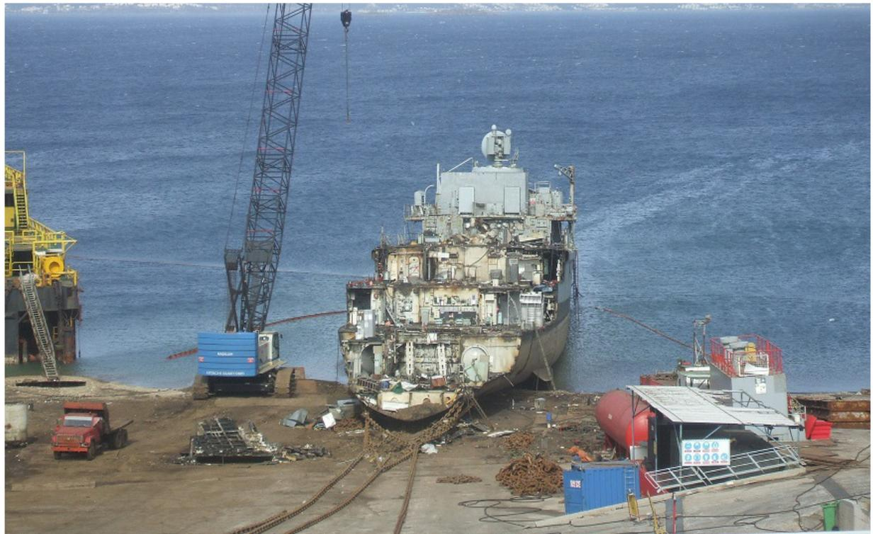
15 Feb 2016 – Ex-HMS York showing the dismantling of the top deck and accommodation. The large blocks removed from the vessel are with the use of heavy lift cranes. Secondary cutting and further processing and material separation takes place.
