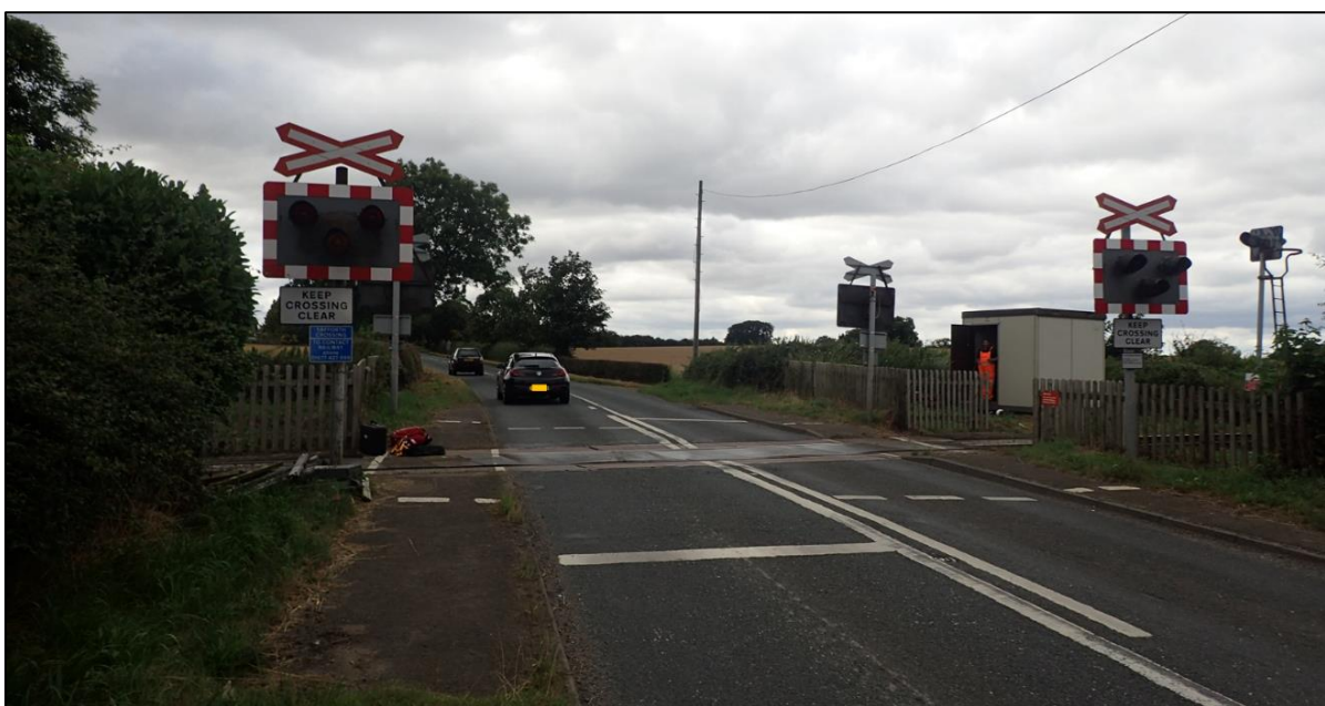
The road traffic signals at Yafforth level crossing for the road approach from the south
