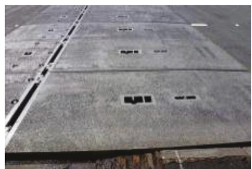
The systems tested by TRL included temporary bridging panels for trenches and excavations up to 2.2 m wide, and a frame with removable concrete filled covers for 2 m x 2 m excavations. Figure 5 shows some examples of the type of plates tested.
