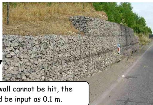
**Fig 5.8-2 Gabion Wall**
