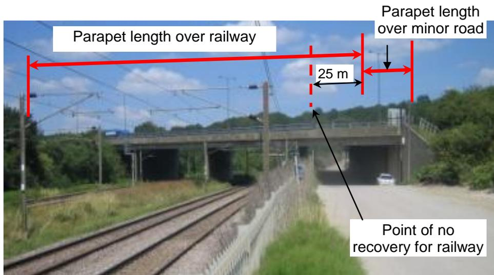
If the lengths in between  $P_{Rail}$  /  $P_{Road}$  / Parapet ends are relatively short, it may be impracticable to have different containment levels from that required at  $P_{Rail}$  and or  $P_{Road}$ . In
