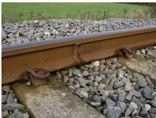
Figure 5.2 Alumino-thermic welded joint
