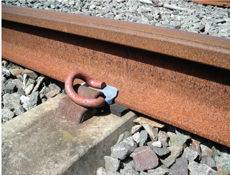
Figure 9.4 Pandrol clip e1809 with BS113A rail on concrete sleepers
