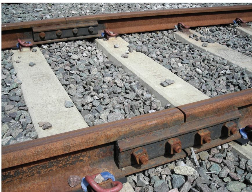
Figure 9.3 Fishplated joint
