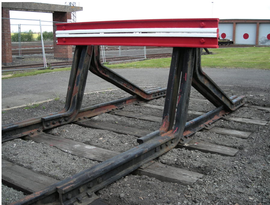
Figure 10.1 Buffer stop
