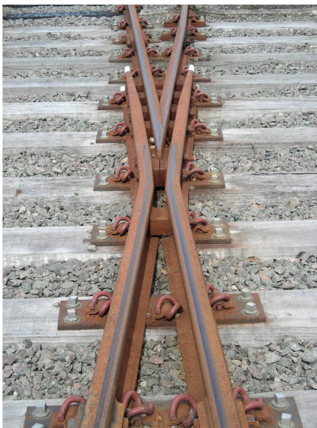
Figure 7.3 Common crossing element within a turnout
