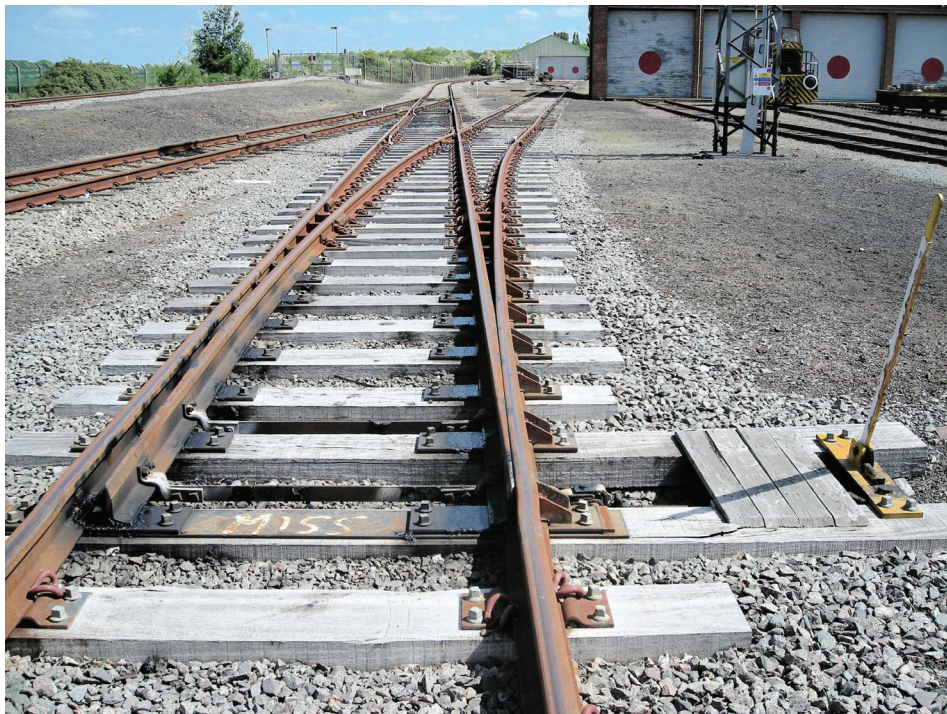
Figure 7.4 Switch element within a turnout
