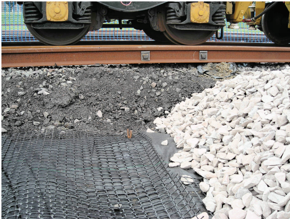
Figure 9.2 Geogrid over geotextile underlaying new bottom ballast
