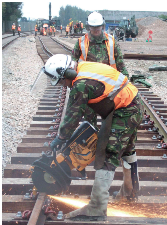
Figure 5.1 Cutting rails by disc cutter
