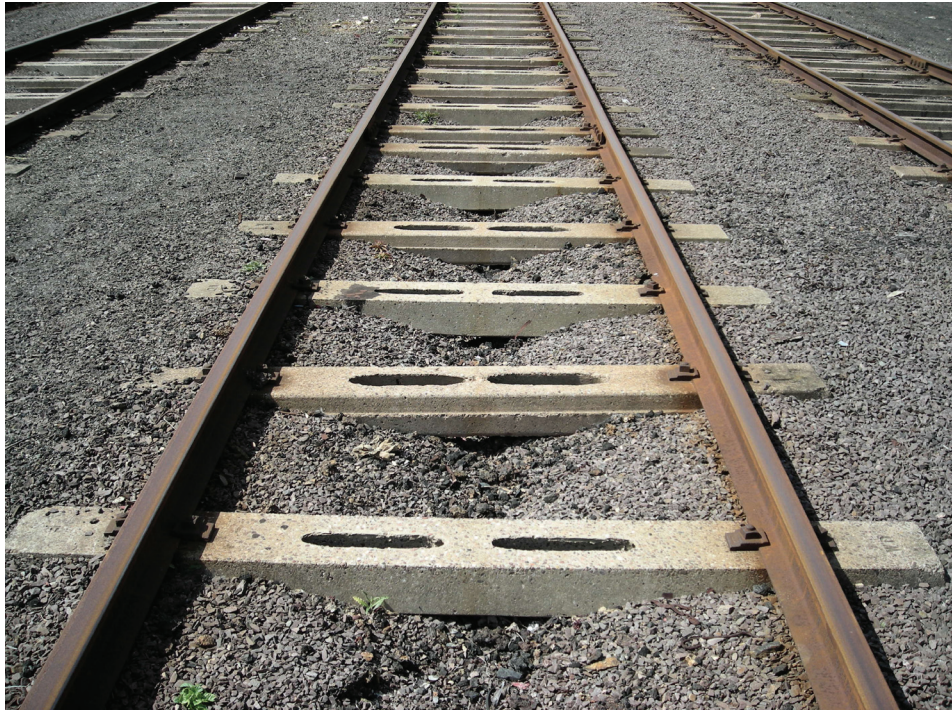
Figure 7.6 Plain line track – obsolete BS75R rail on concrete sleepers
