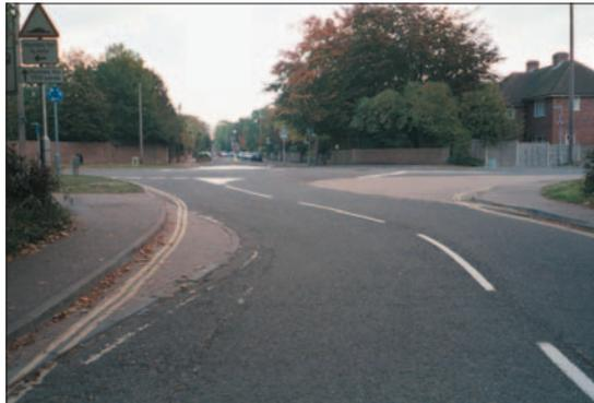
Photo 4.2.9: Mini-roundabout with overrun area
