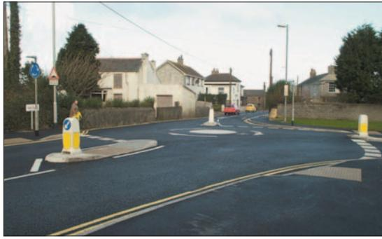
Photo 2.3.2: After view of junction with mini-roundabout
