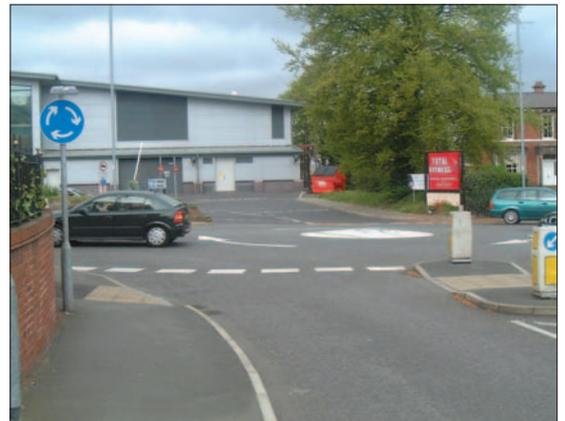
Photo 2.6.1: Mini-roundabout as access to new development
