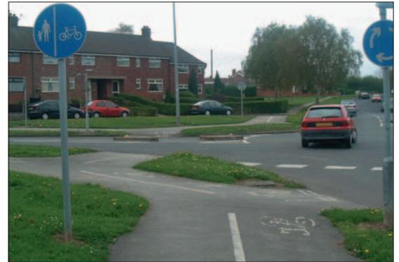
Photo 3.11.2: Mini-roundabout with off-highway cycle facilities
