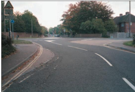
Photo 4.2.9: Mini-roundabout with overrun area
