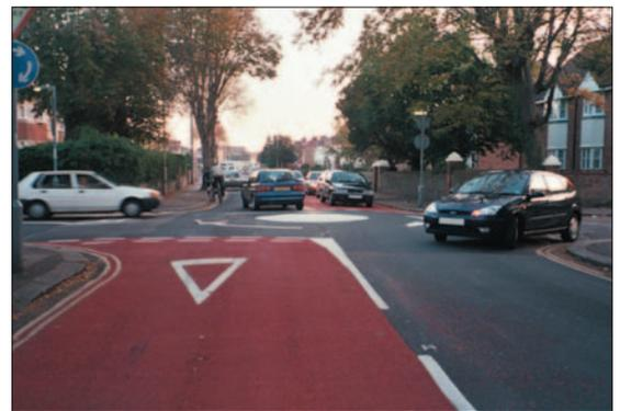
Photo 4.2.10: Mini-roundabout with red anti-skid
