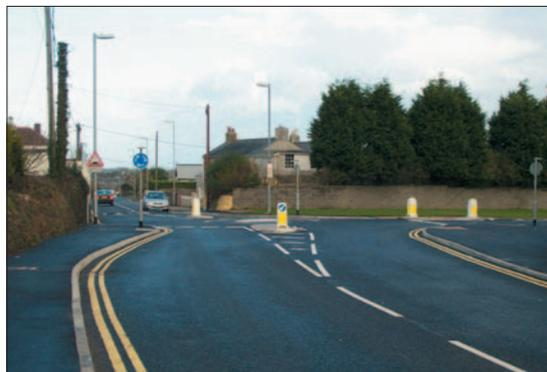
**Photo 4.2.4: Deflection through alignment and traffic island**
