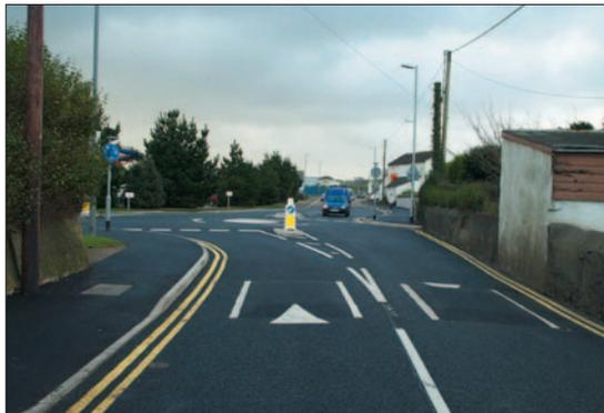
**Photo 3.13.4: Traffic calming on approach to mini-roundabout**
