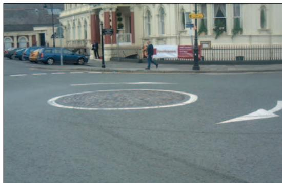
Photo 2.1.6: Non-conforming central marking in setts with white edge marking
