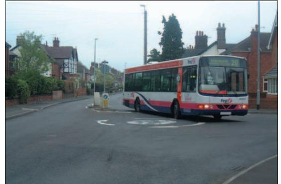
Photo 3.13.1: Bus at mini-roundabout with severe deflection
