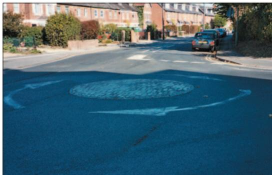
**Photo 4.5.2: White paint wearing on blockwork central island**
