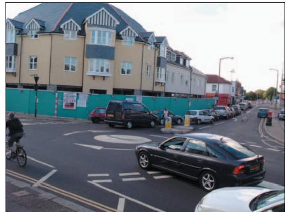
**Photo 3.7.4: Mini-roundabout near level crossing**
