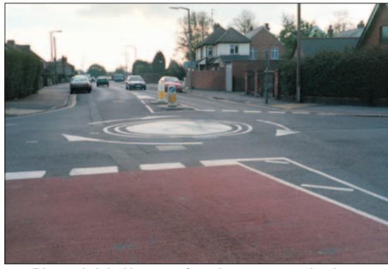
**Photo 2.1.3: Non-conforming concentric rings**
