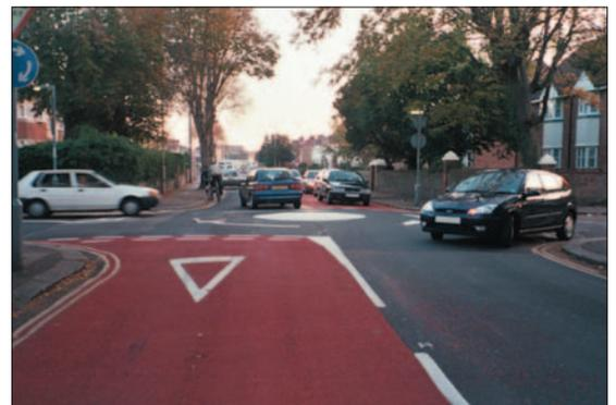
Photo 4.2.10: Mini-roundabout with red anti-skid
