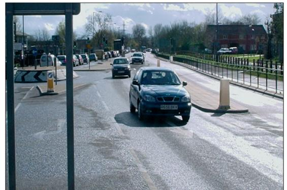
Photo 3.13.2: Bus bypass at 3-arm small roundabout shows a similar application
