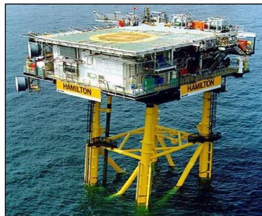
These platforms are two-level, normally unmanned structures with an underdeck. Produced gas, together
