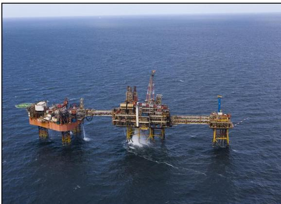
The layout of the Douglas Complex is designed with the objective of separating the potentially hazardous production plant and well facilities from the living quarters and control centre. The three platforms are orientated to provide the smallest target to passing ship movements. Water depth at the location is 29 metres.
