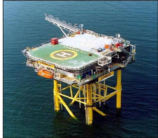
Lennox produces both gas and condensate, together with formation water. These reservoir fluids are routed to the Douglas Complex for separation. Lennox lies approximately 8 km off the Sefton coast. The Lennox Platform is a two level, 12 well slot structure with an underdeck. Water depth at the location is 7m.
