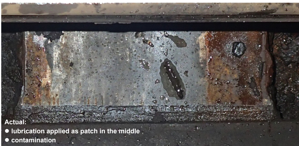
Figure 9 – Switch rail to baseplate interfaces (representative examples)
