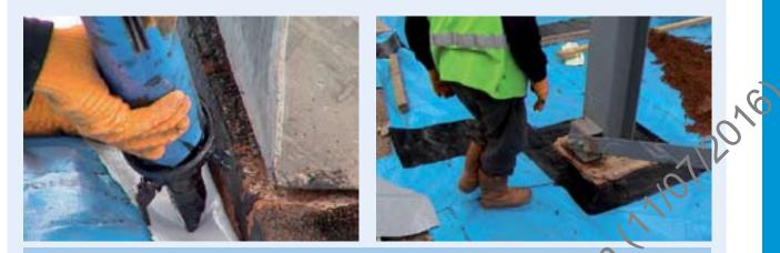
Make sure the root barrier membrane is sealed properly around pillars and other sure tures.
