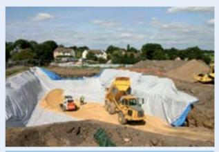
**Stage 4:** Protect the root barrier membrane from tyre damage with a layer of sand.
