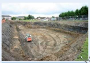
Stage 1: Calculate volume required and excavate site, allowing for 2m depth of burial
