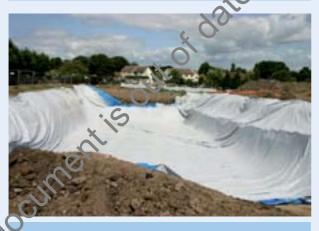
**Stage 3:** Put root barrier membrane in place, allowing enough material along the edges to eventually provide a seal.
