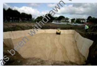
**Stage 2:** Protect the integrity of the root barrier membrane with a layer of sand and provide shutter ply supports for the edge of the cell.
