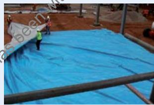
**Stage 1:** Protect the integrity of the root barrier membrane and prevent dama room 'heave' with a layer of sand.
