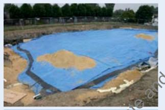
**Stage 7:** Put the surface of the root barrenembran in place and make sure the cell is adectately sealed.
