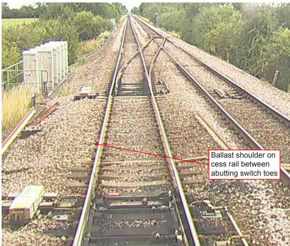
Figure 12: Ballast shoulder in plain line section between 102A and 101B points, captured by the forward facing CCTV camera on Network Rail's track recording train, August 2014 (image courtesy of Network Rail)
