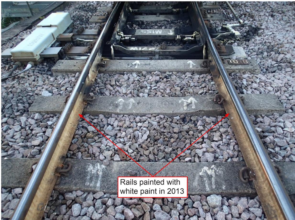
Figure 11: Sleeper tops above ballast at toe of 101B points
