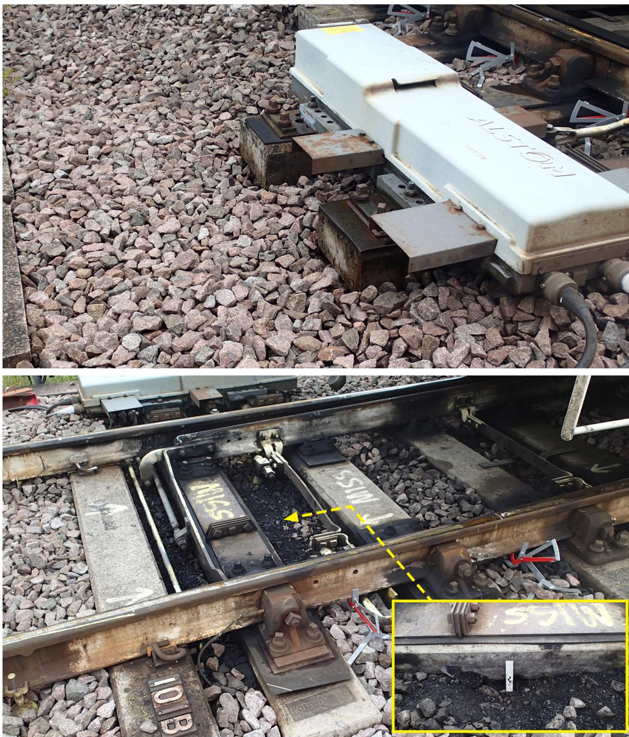
Figure 9: Ballast support at the ends of 101B point motor bearers and in the 'cribs' at the toe of the points
