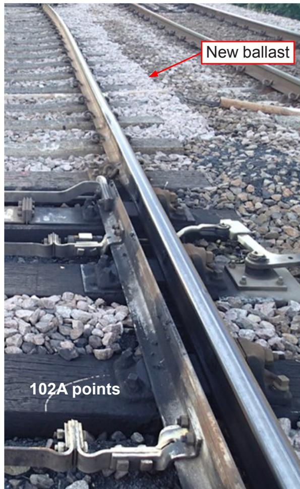
Figure 13: Area of ballast dressing in the six-foot between 102A and 101B points
