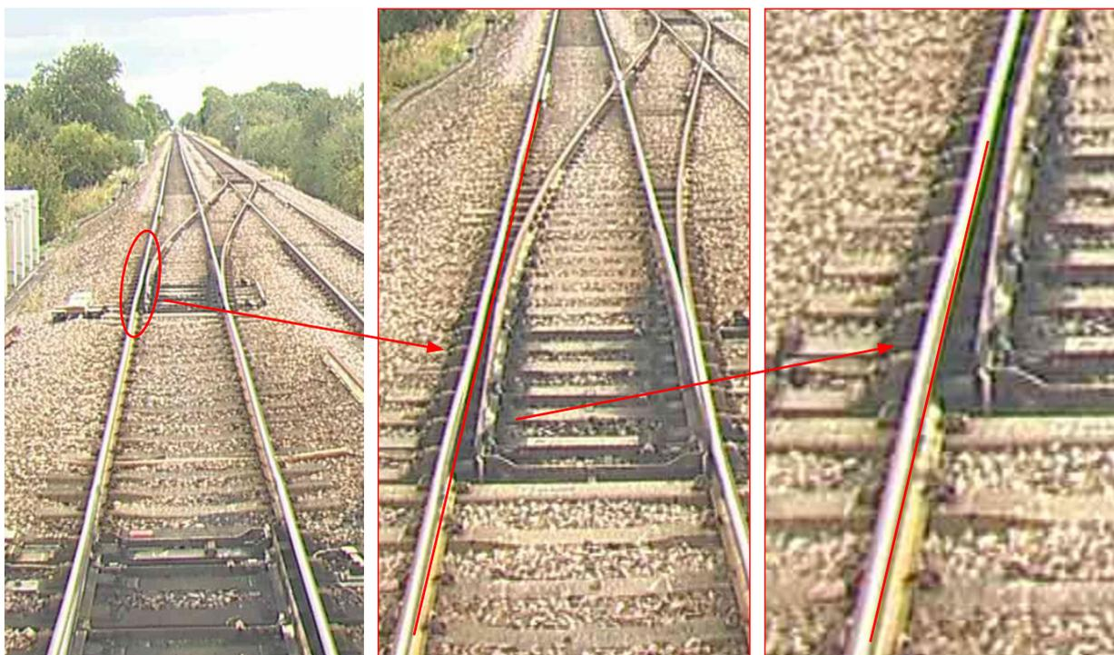
Figure 14: Pre-existing misalignment on LH rail at 101B toes, captured by the forward facing CCTV camera on the Network Rail's track recording train, August 2014 (image courtesy of Network Rail)
