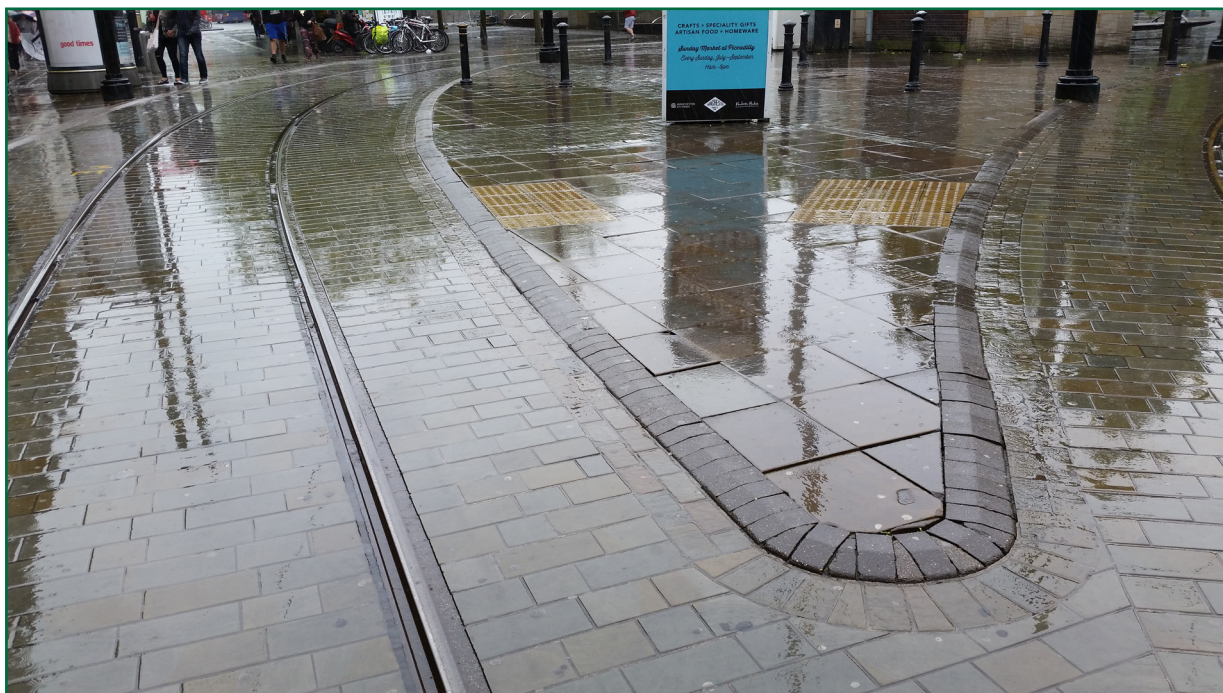
Figure 7: Demarcation of tramway (view in opposite direction from figure 5)
