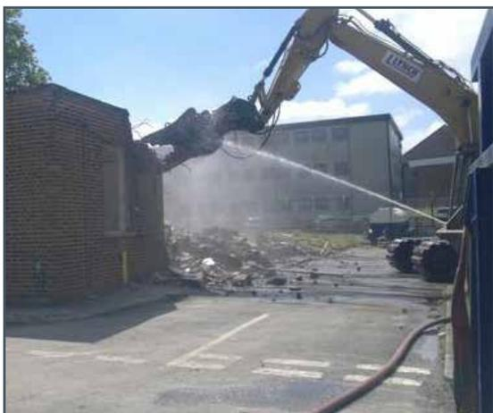
Demolition of former liquid effluent treatment plant buildings in 2015.
