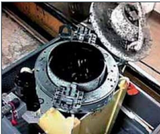
Sludge canisters being removed from the Berkeley vaults.
