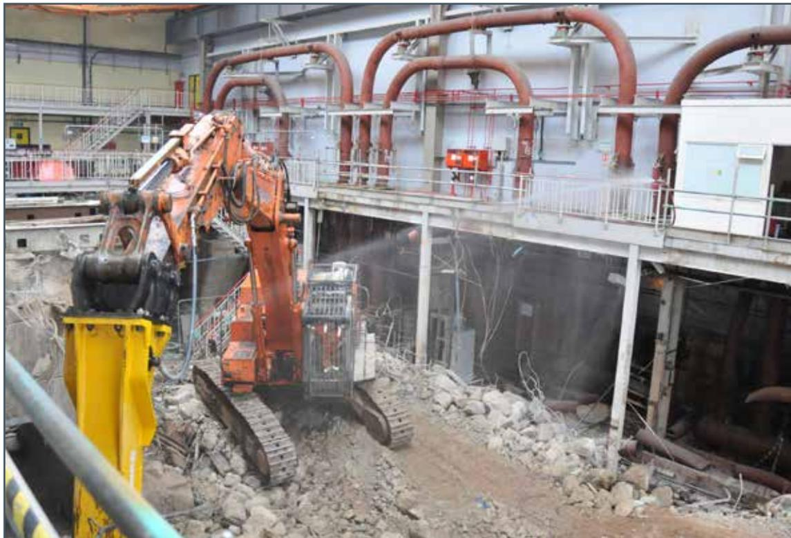
**Demolition of the auxiliary turbine hall at Bradwell, with dust suppression implemented through water sprays.**
