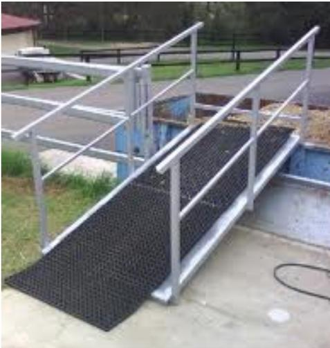
This photo shows the use of a portable ramp system used in a change of level
