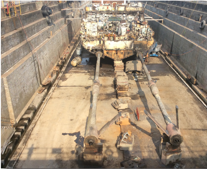
Final stages of dismantling in the dry dock.
