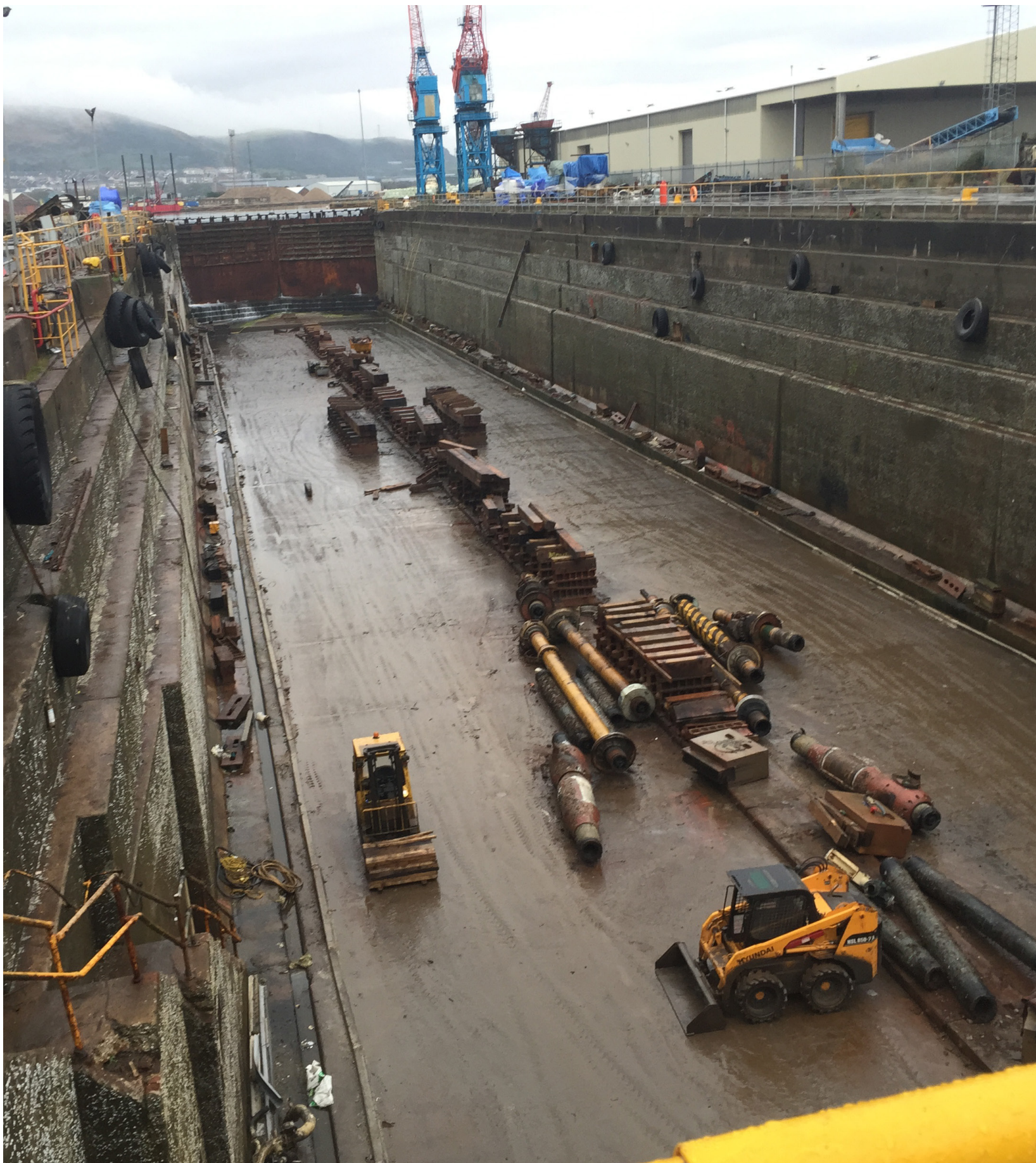
The final Pictures of the dry dock where the Former HMS Cornwall was dismantled. The final pieces were removed from dry dock no.2 on the 30th October 2014 twelve months to the day of her arrival. Thorough cleaning of the dock is undertaken prior to re-flooding in preparation for the next ship arrival.
