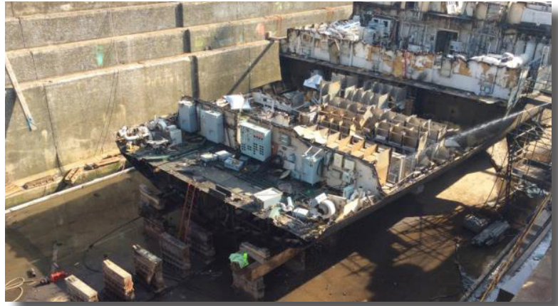
Various stages of dismantling in the dry dock of the superstructure Sept 2014.
