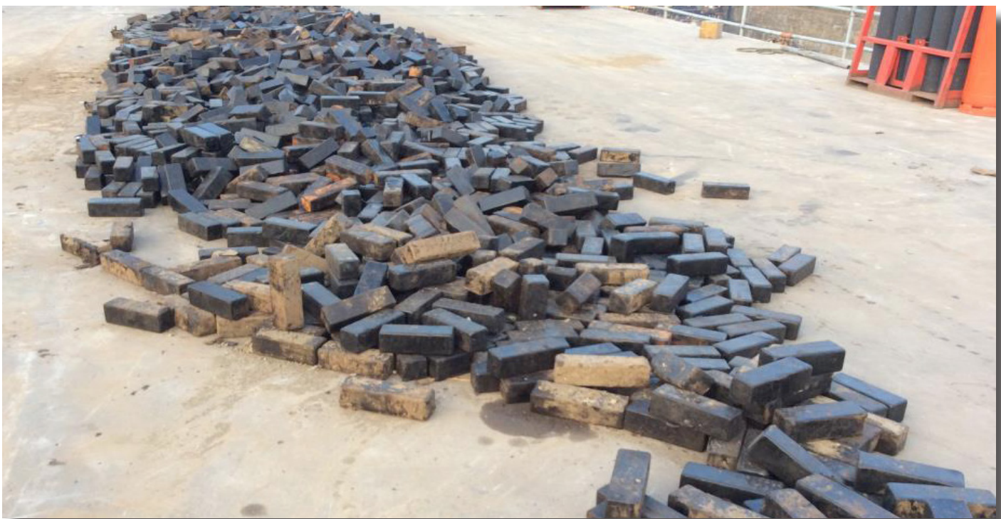
Lead Ballast Aug 2014 182 tonnes removed in total.
