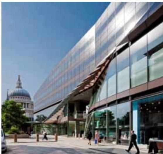
The building's green credentials are enhanced by solar-controlled glass, limiting heat gain to reduce the need for air conditioning.
