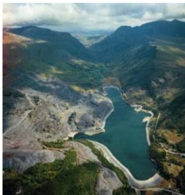
An overhead view of Dinorwig's lower reservoir, Llyn Peris
