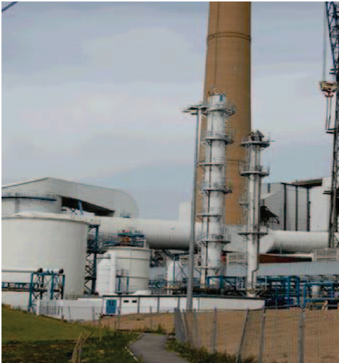
The CCPIlot100+ capture project at Ferrybridge power station.
