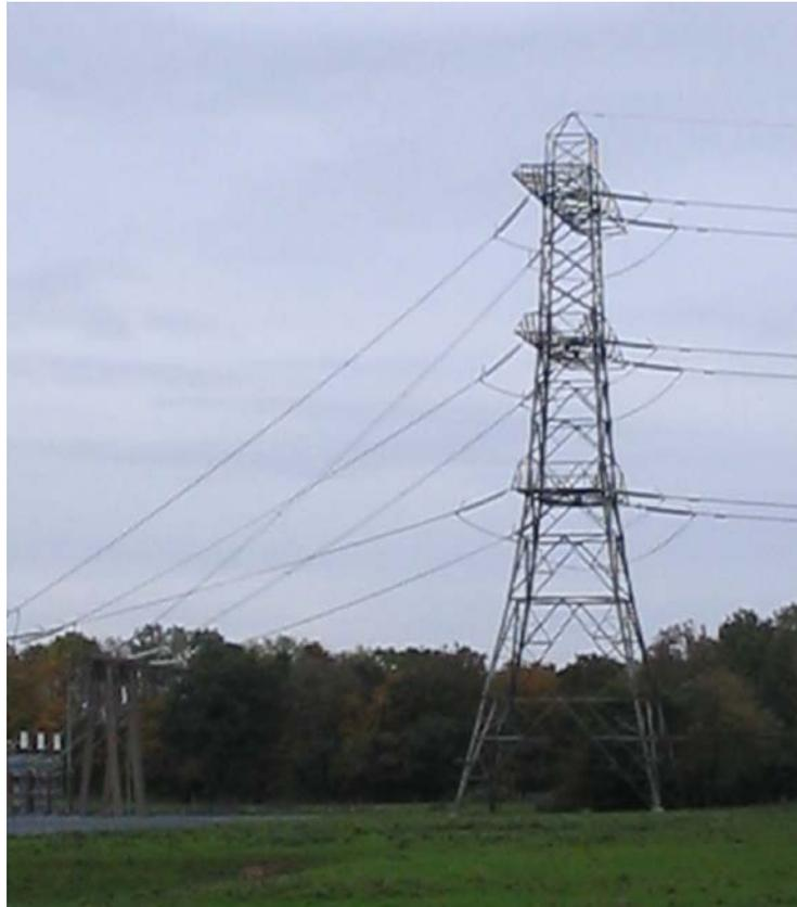
The order of these downleads determines the phasing of the line. It will normally be reasonable for the electricity industry to achieve optimum phasing for high voltage power lines when it can be done by means of reconfiguring these downleads. This would apply to new power lines and to the conversion of existing power lines.
