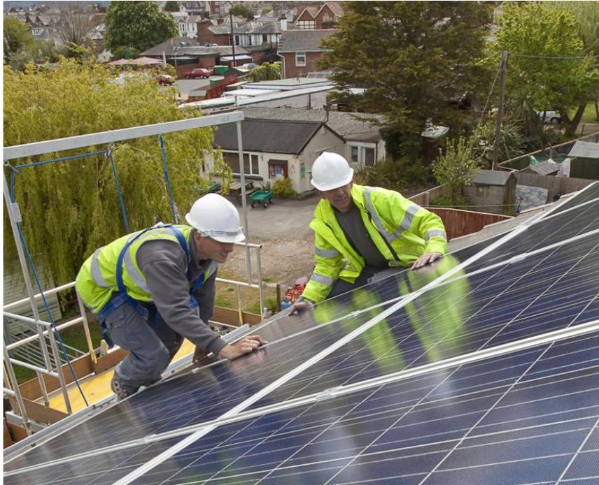
*Installers at work fitting solar PV panels on a roof*
