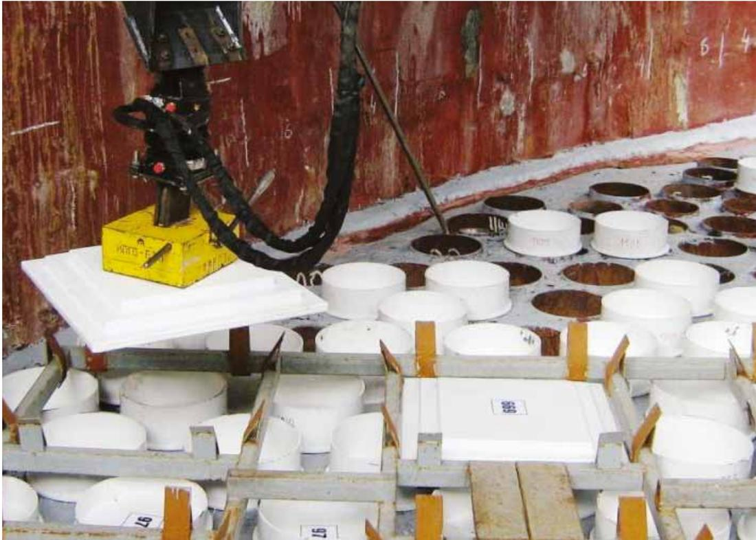
Installation of the biological shielding over SNF in DSU 2A at Andreeva Bay, NW Russia.
