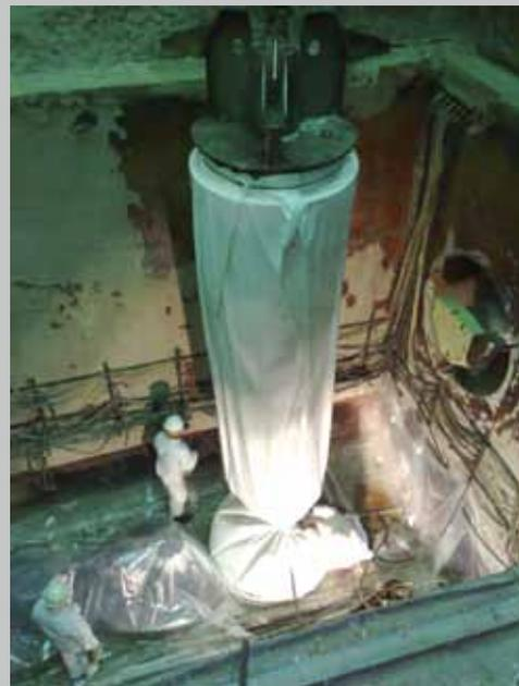
Removal of an Intermediate Heat Exchanger for examination of the effect of carbonation from passivation of the primary cooling circuit at BN-350.
