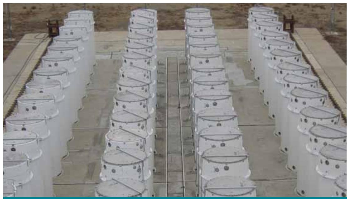
Fuel from the decommissioned plutonium-producing BN-350 nuclear power plant at Aktau, Kazakhstan, in a safe and secure storage facility at Semipalatinsk.
