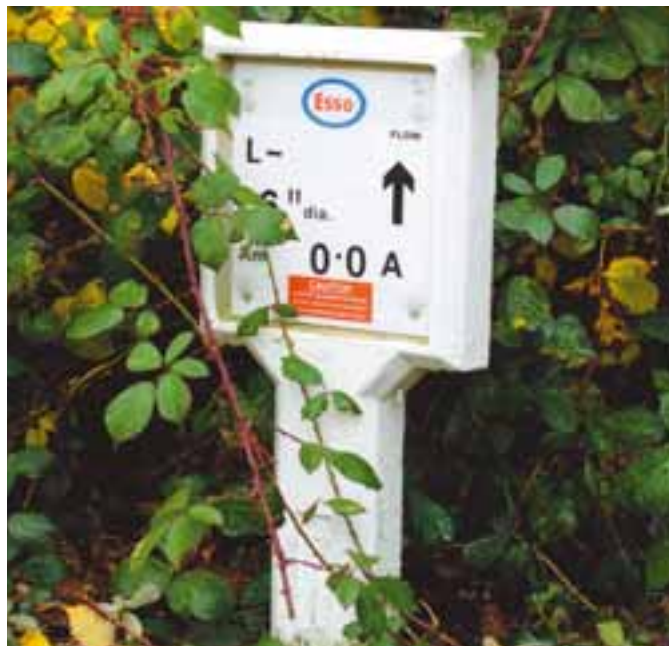
Oil pipeline marker post.
