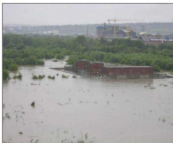
Photograph 11 - An electricity substation protected by flood barriers in the 2007 floods in the North East of England
