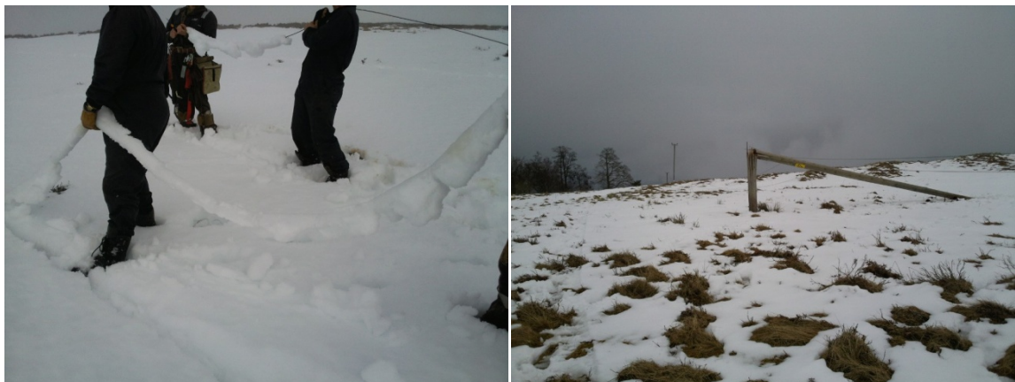
Photograph 4 - The effect of icing on an 11,000 volt rural overhead line in North West England in January 2010
