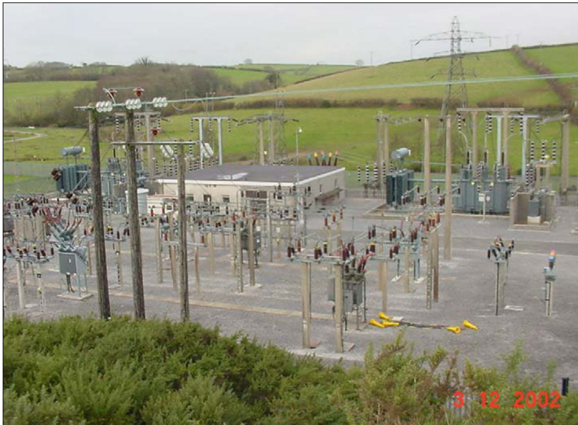
Photograph 9 - 132kV Grid Substation showing 132kV terminal tower (pylon) and start of 33kV wood pole overhead line.
