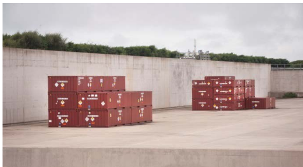
LLW containers in engineered vaults at the repository
