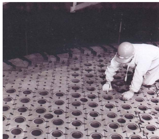
Reactor core graphite
